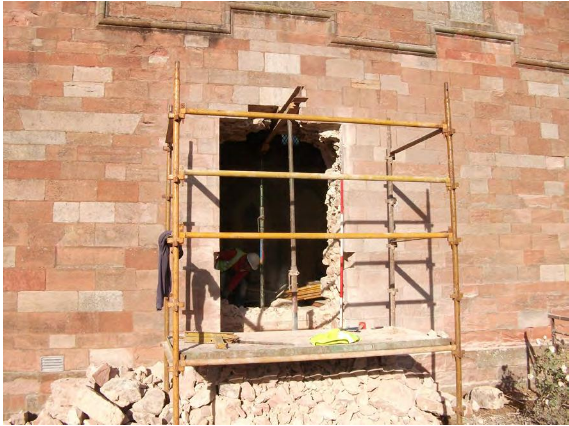
Fig.9 : Completed door slapping from the exterior
