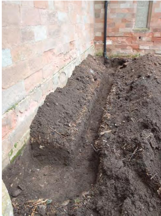
Fig.13 : Drainage trench
