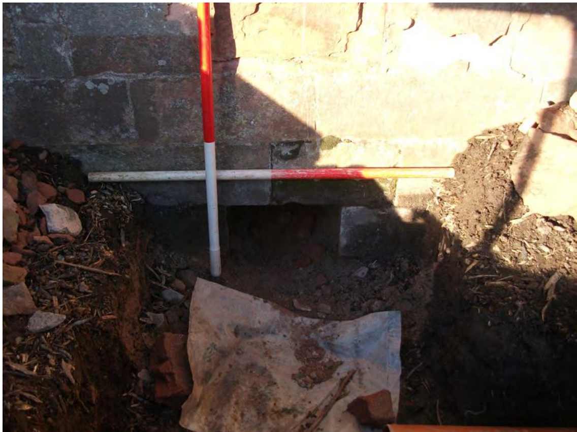
Fig.12 : External elevation showing slapping for drainage pipe
