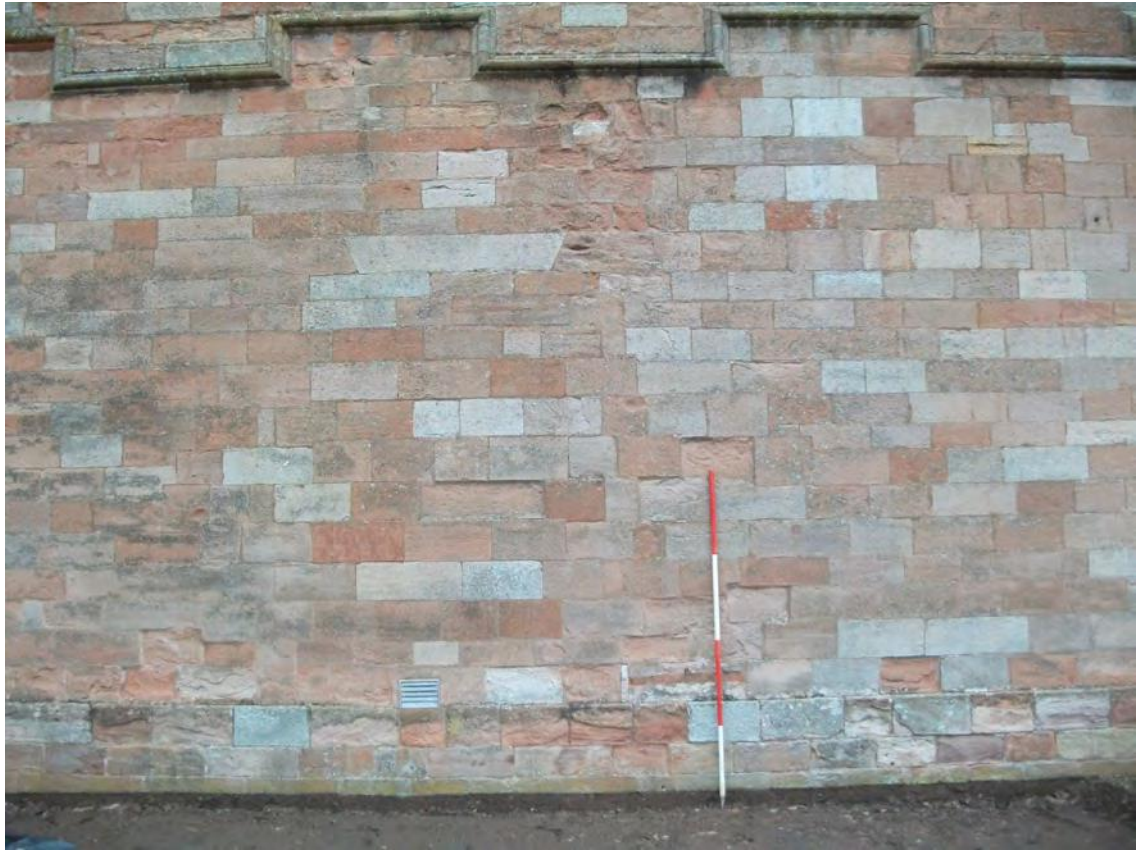
Fig.3 : South-facing external elevation prior to new door slapping
