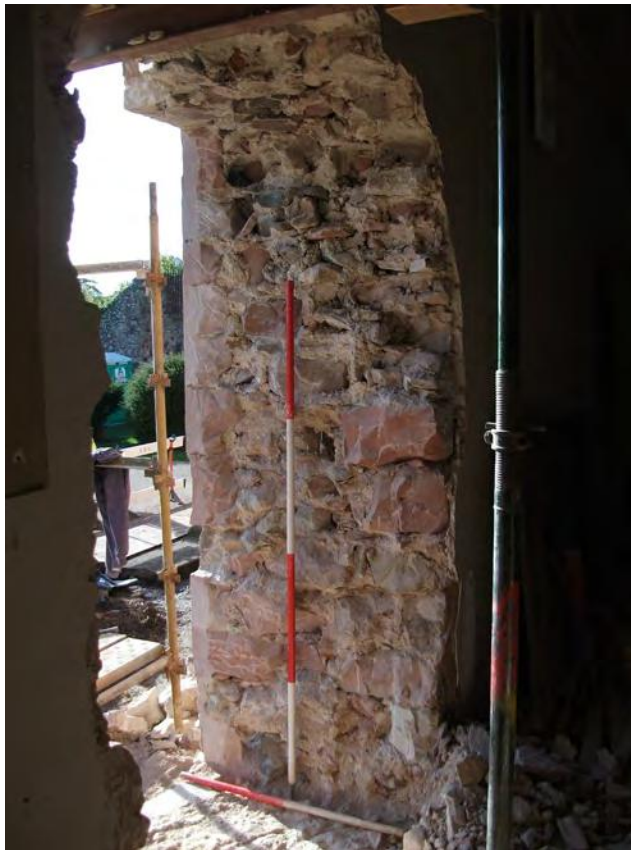
Fig.7 : East-facing section of new door slapping
