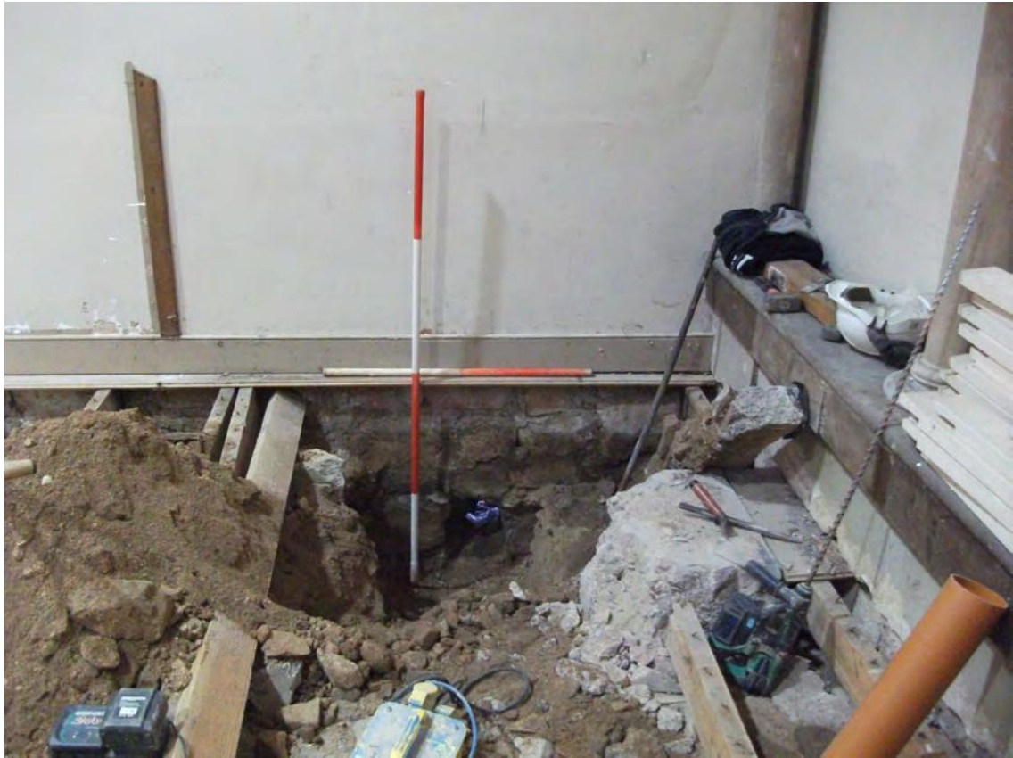
Fig.11 : Internal elevation showing slapping for drainage pipe
