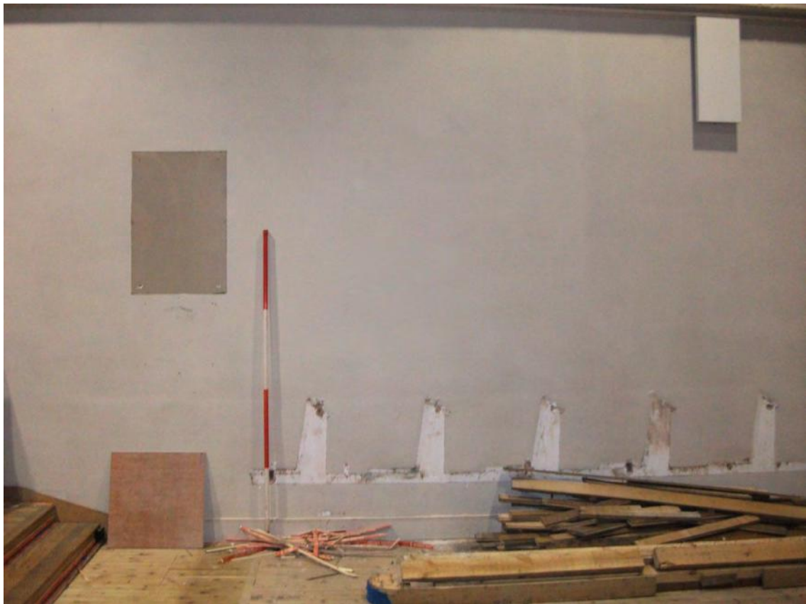
Fig.4 : North-facing internal elevation prior to new door slapping
