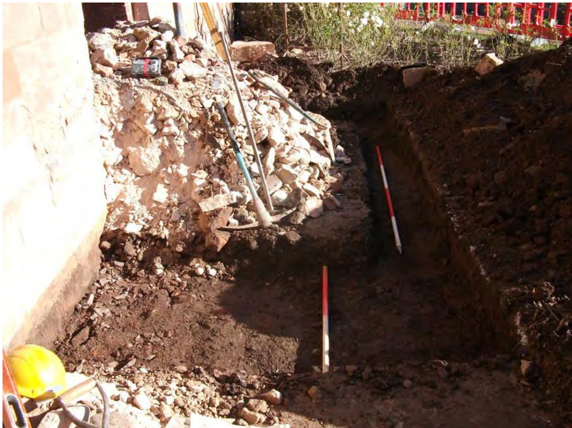
Fig.16 : Foundation excavations for platt
