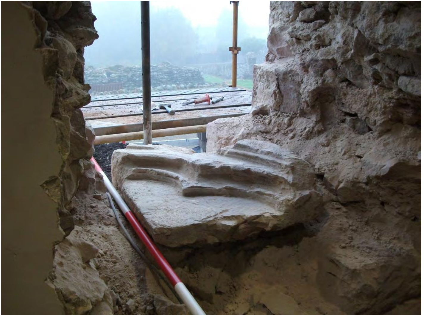
Fig.5 : Large masonry sedilia fragment in situ within wall
