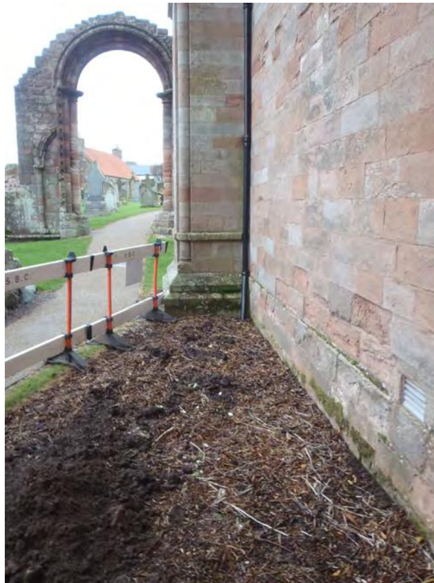
Fig.10 : South-facing external elevation prior to slapping for drainage pipe
