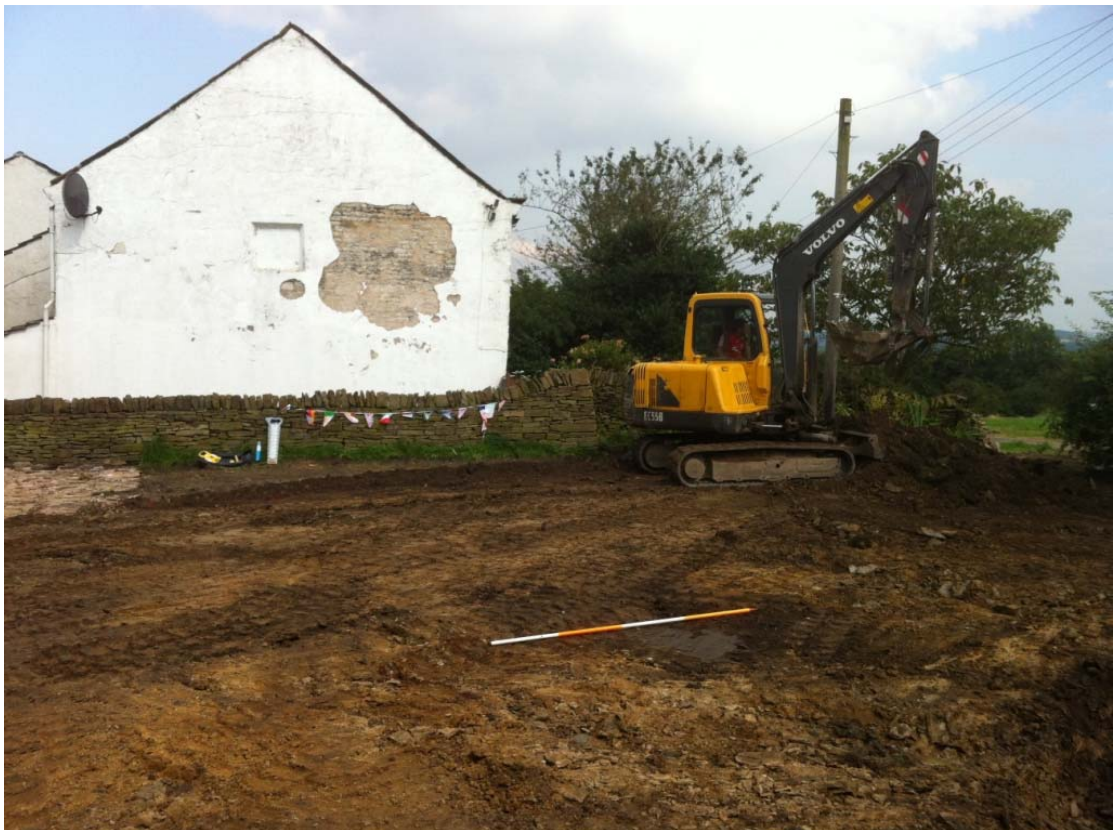
Plate 2: Working shot showing the watching brief area, looking north-east
