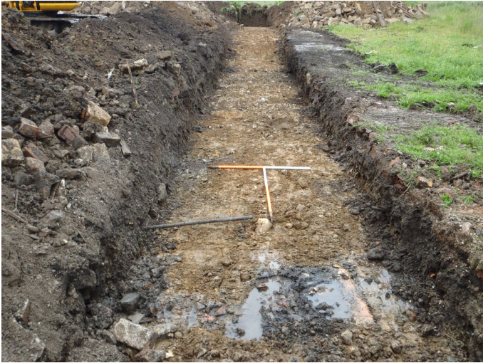
Fig. 3 - Trench H from the east
