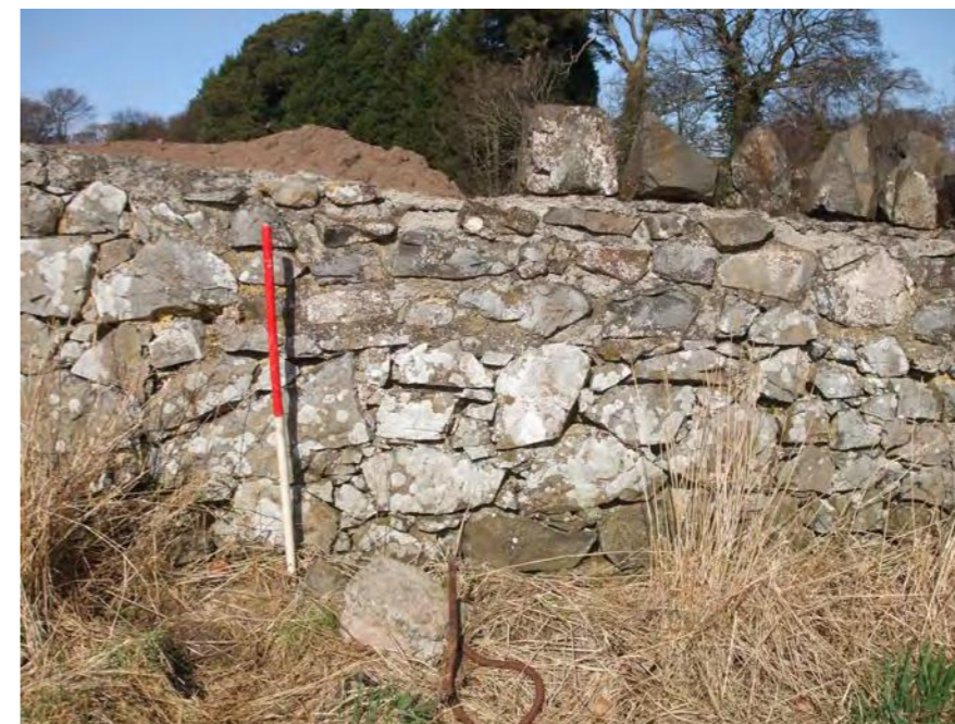
Fig. 10 - Wall 2, general shot from S prior to demolition
