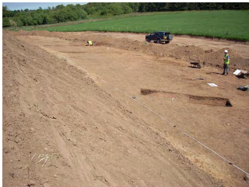
Fig. 5 - General shot of Site 1
