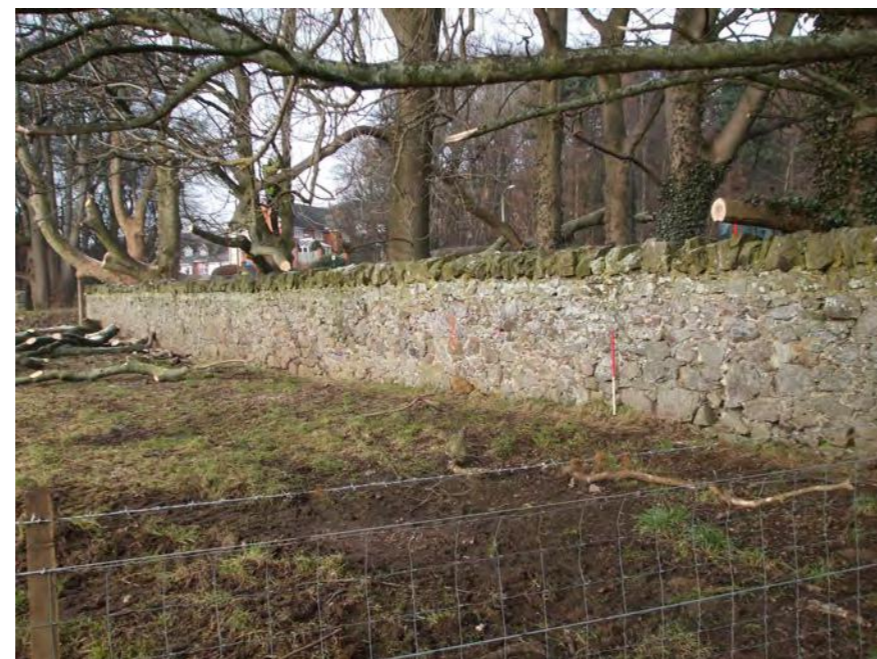
Fig. 9 - Wall 1, general shot from SE prior to demolition
