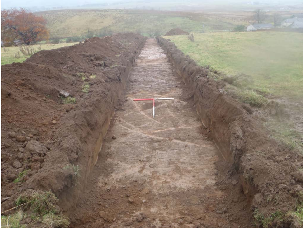
Fig.4 : Trench 38 from the north west
