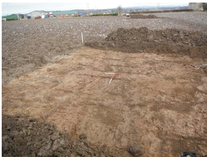
Fig. 3 - Turbine Base 2, looking E
