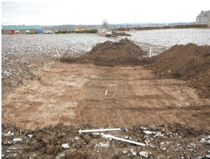
Fig. 2 - Turbine Base 1, looking E
