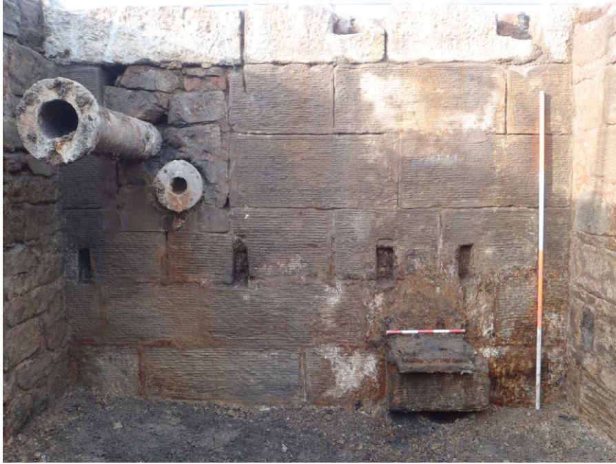
Plate 27. Elevation 5003, Room 1, Structure 5
