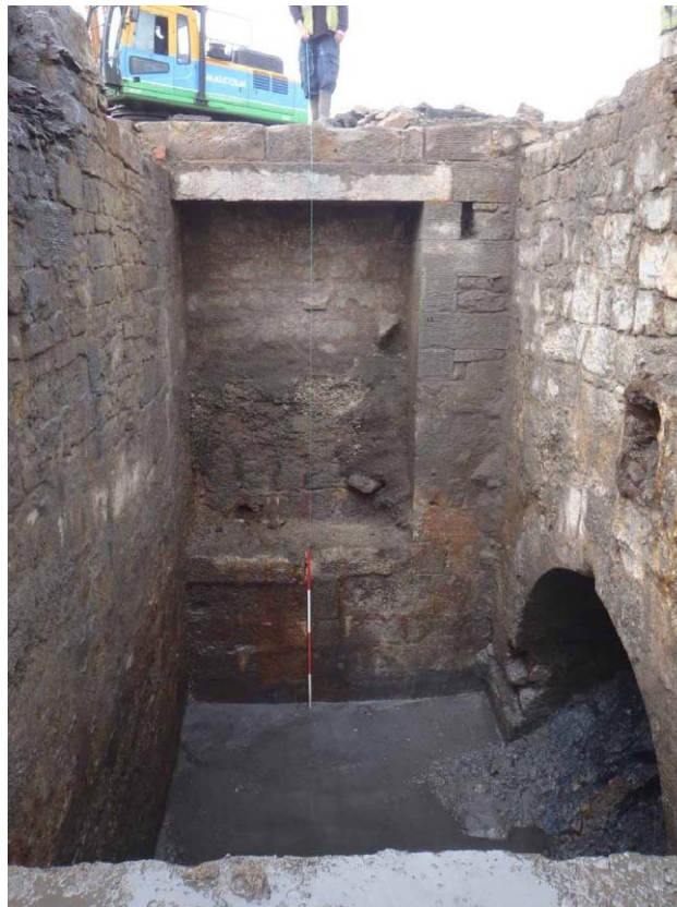
Plate 26. Internal south-west facing elevation, blocked opening and masonry arch in Room 1, Structure 5
