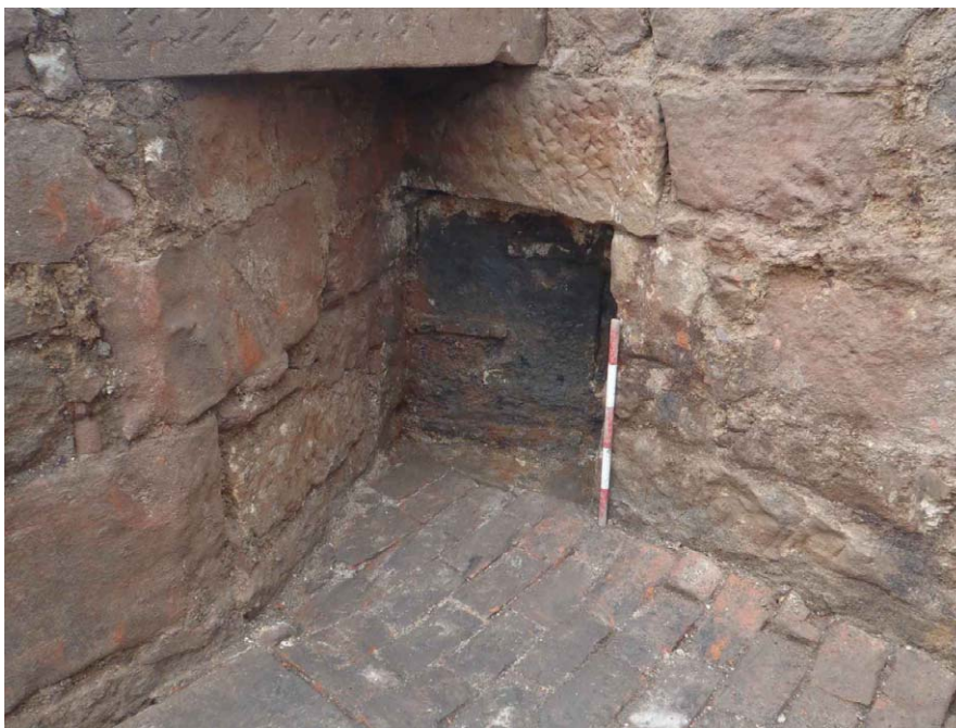
Plate 34. Boiler House outlet with cast iron door, Structure 8
