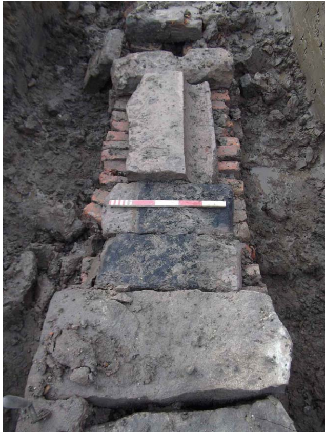
Plate 39. Brick culvert 3022 and sandstone capping (3021), Structure 3
