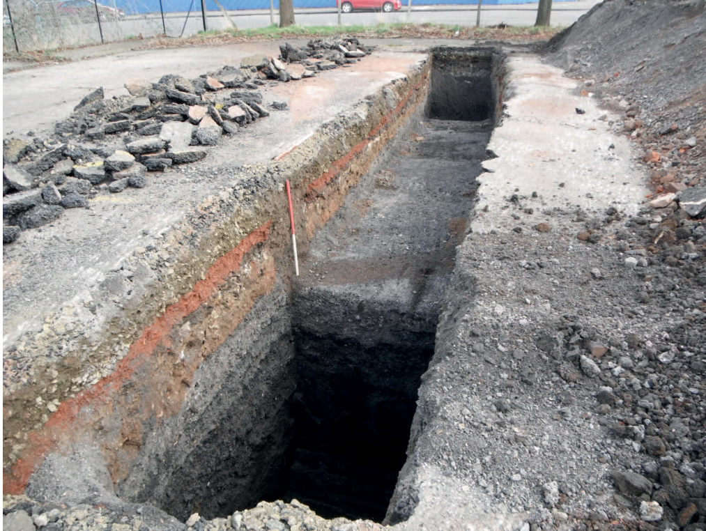
Fig.7 Trench 2 looking north-east
