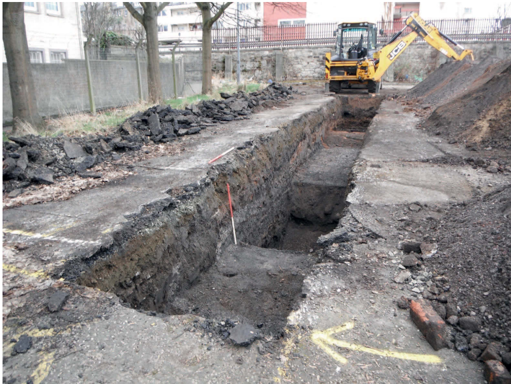
Fig.6 Trench 5 looking south-west
