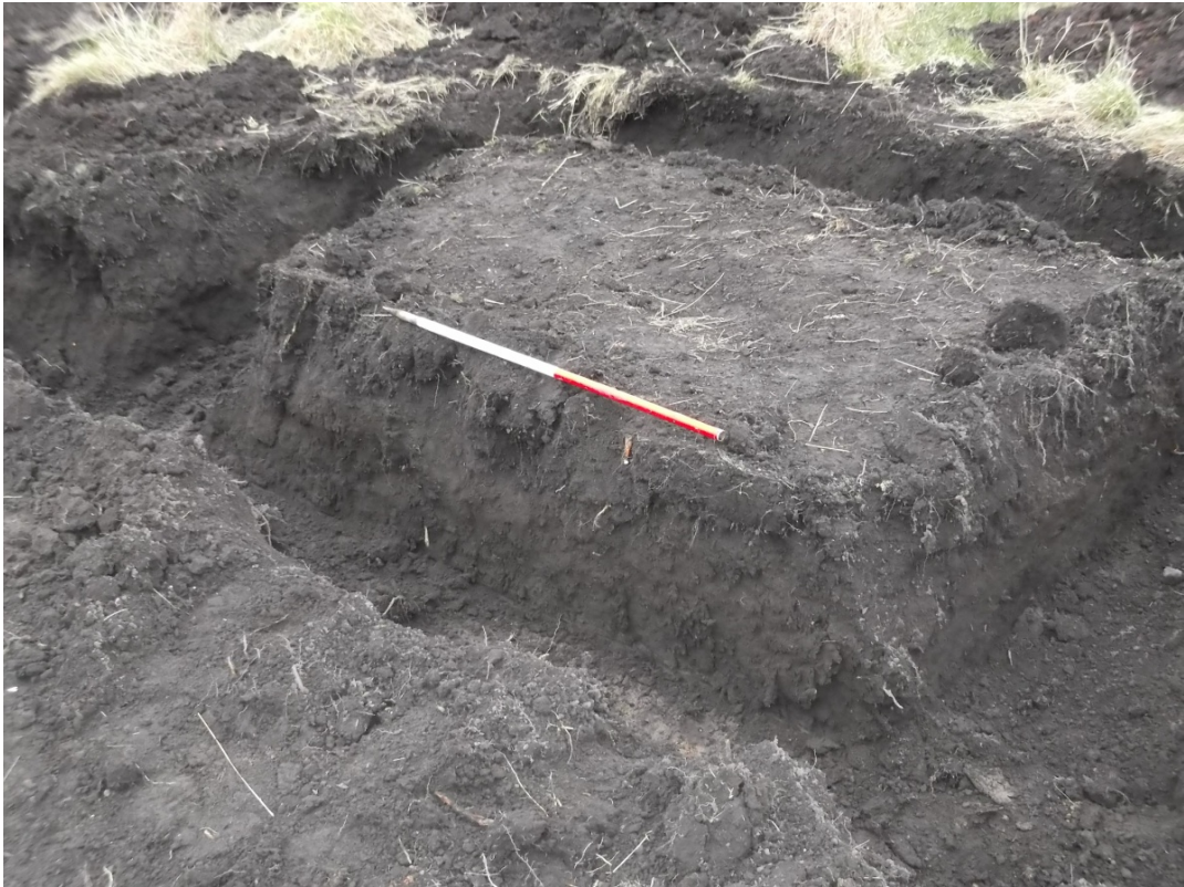
Plate 1: Building A; foundation trench post-excavation, shot facing northwest
