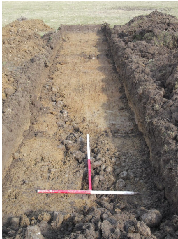
Fig. 5 - Post-excavation shot of Trench 8 showing stone field drain
