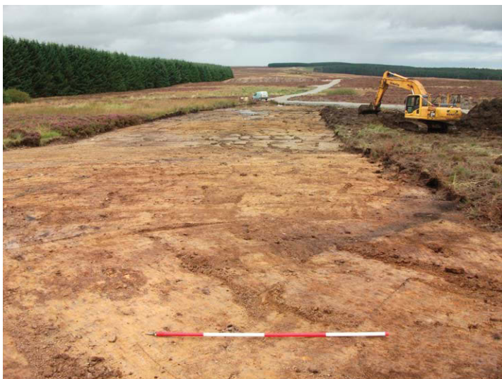
Fig. 7 - Shot of Turbine 9 after topsoil removal
