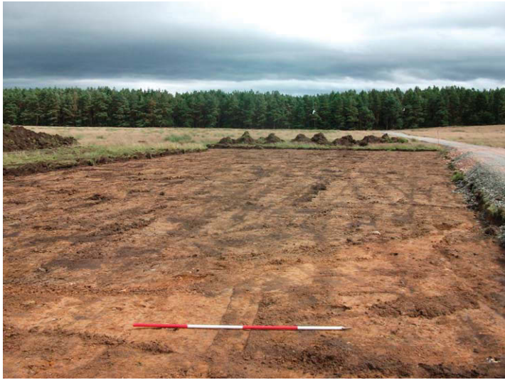
Fig. 9 - Shot of Turbine 1 after the removal of topsoil
