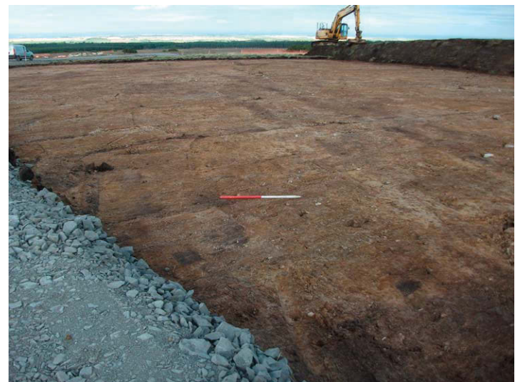
Fig. 8 - Working shot of topsoil removal at Turbine 4
