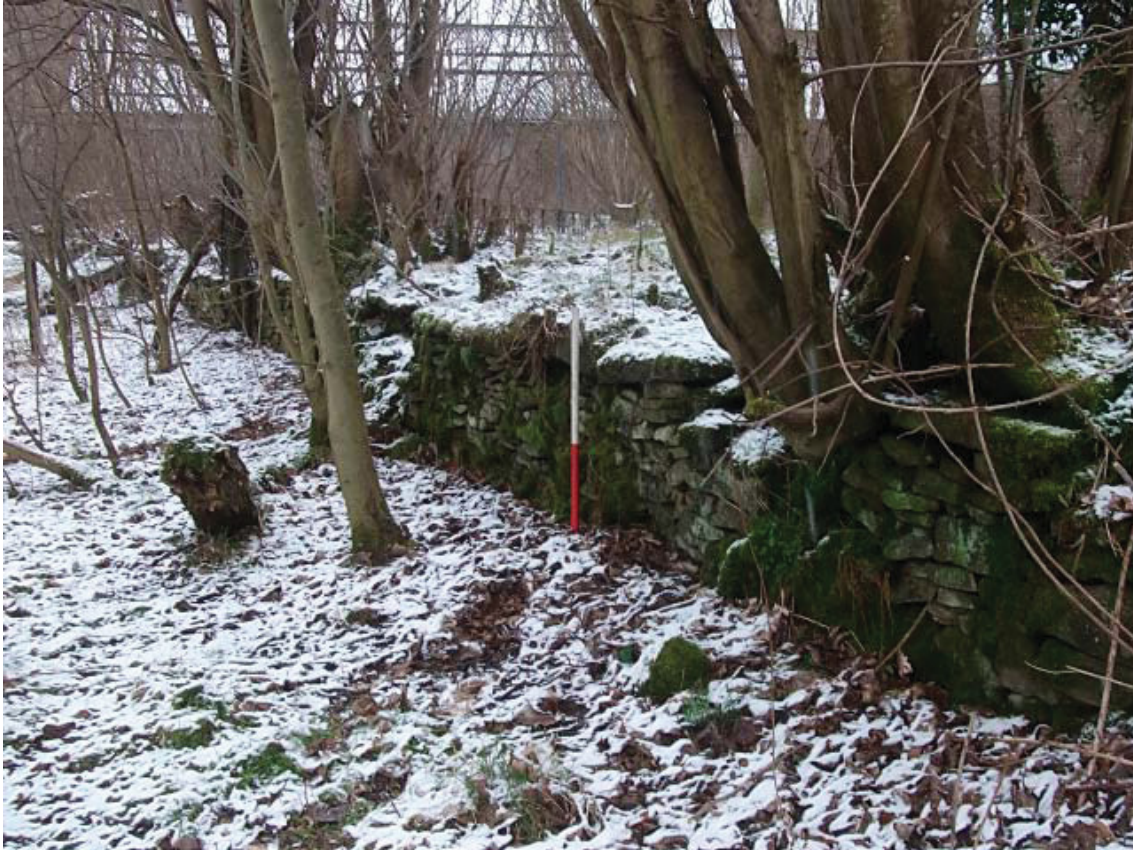
Plate 1 - Upstanding north-west-facing interior reservoir wall at east of development
