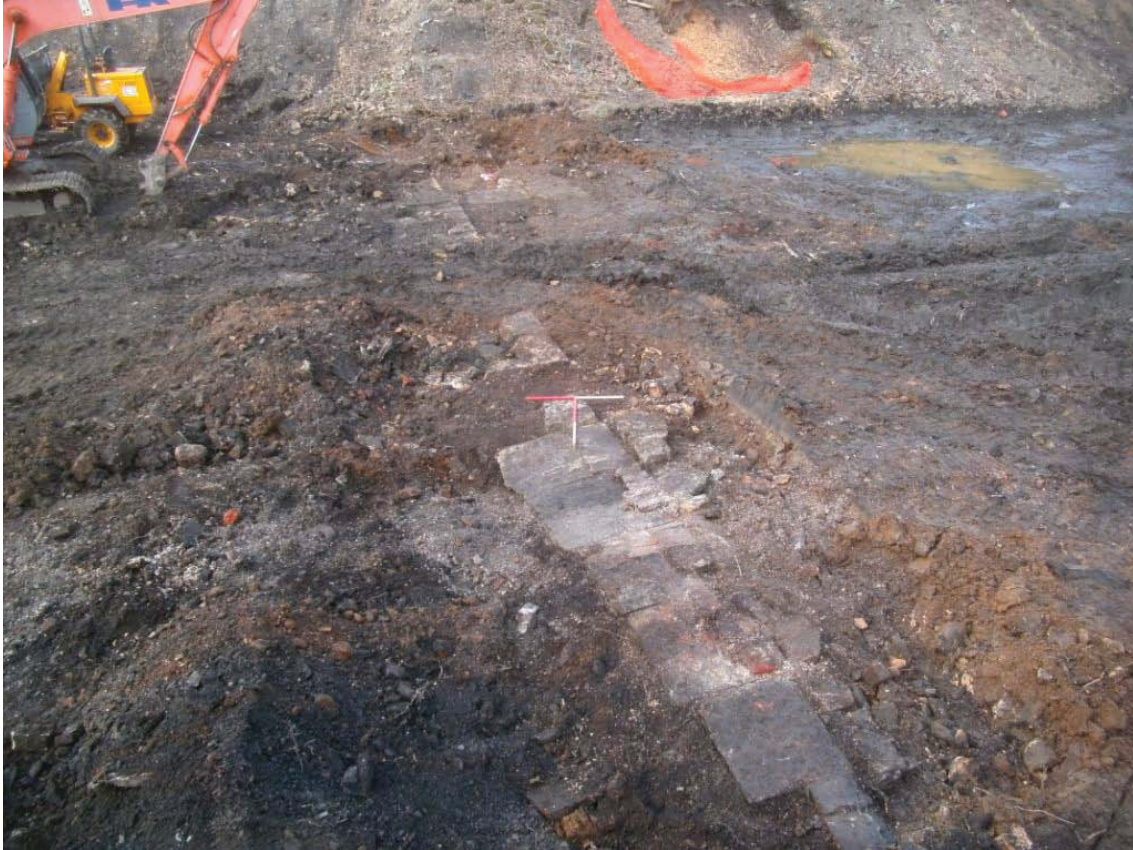
Plate 3 - Shot of western exterior wall of reservoir showing paved surface 010
