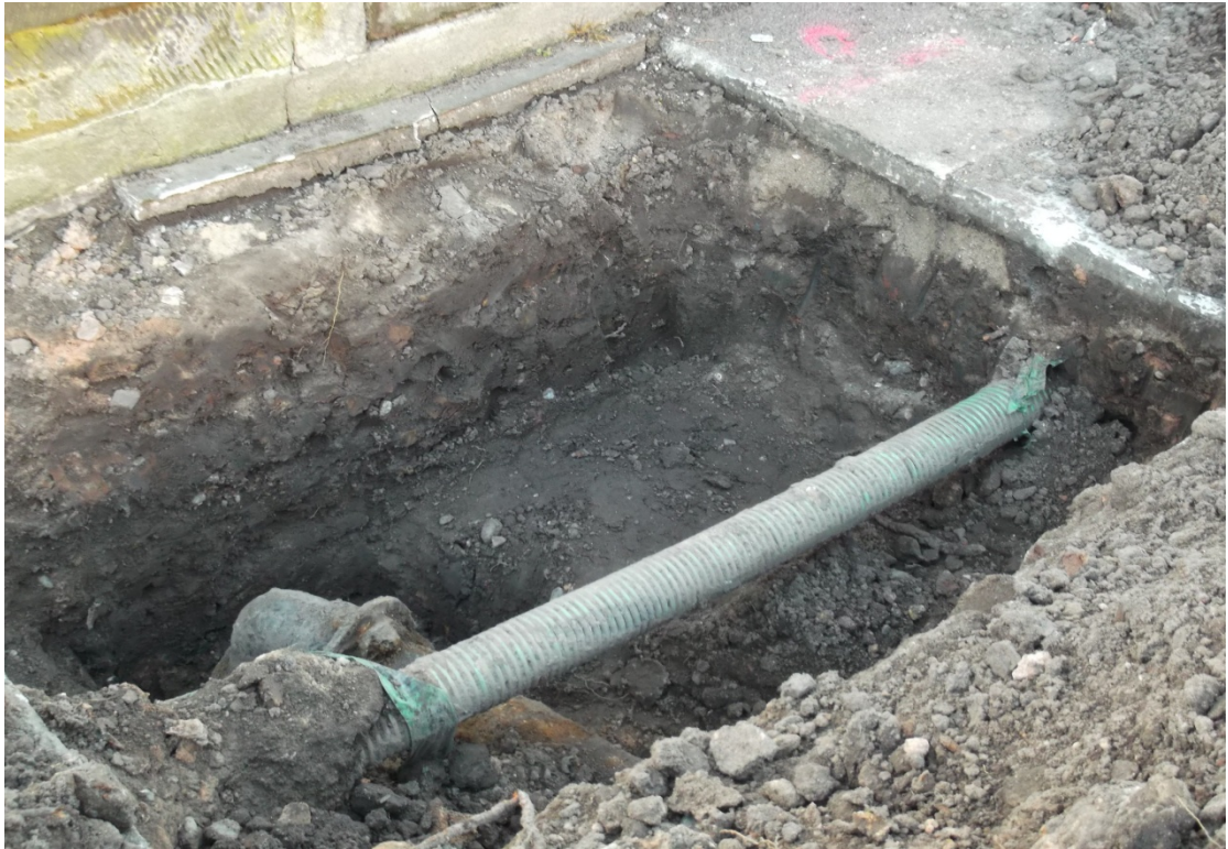
Plate 1: Test Pit 2 access trench fully excavated, shot facing east
