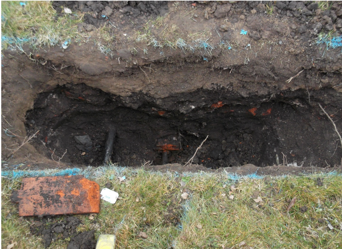
Plate 3: Test Pit 1, east facing section showing demolition layer 102 and exposed services
