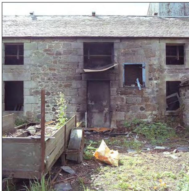
Plate 13 - Range A, North elevation, blocked doorway and open windows.
