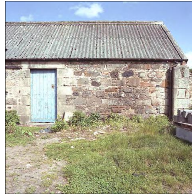
Plate 27 - Range D, South elevation east end. The remains of an entranceway to the demolished East Range is visible at right of picture.
