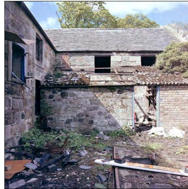
Plate 18 - Range A and B with asbestos roofed pig-sty.
