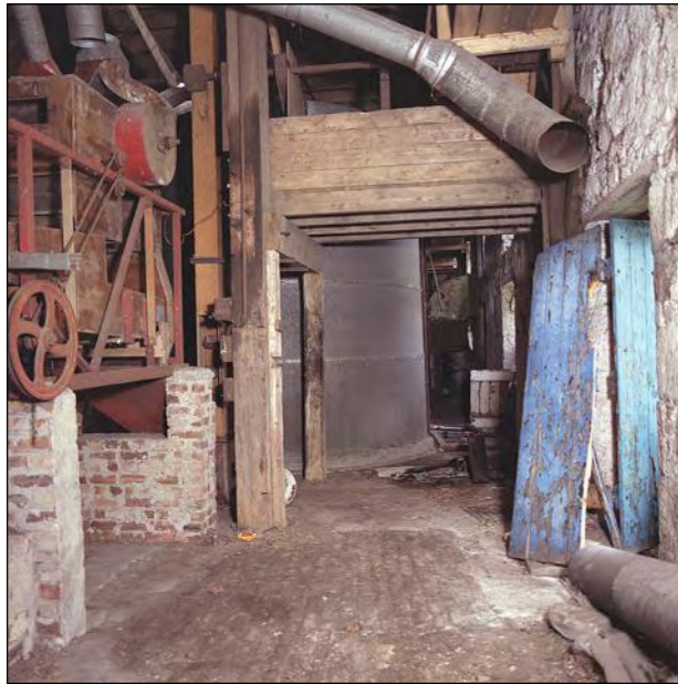
Plate 49 - Range A, Interior detail of the grain silos machinery, looking west.
