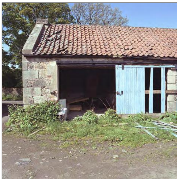
Plate 21 - Range C, East elevation of tack-room and stable entrance.
