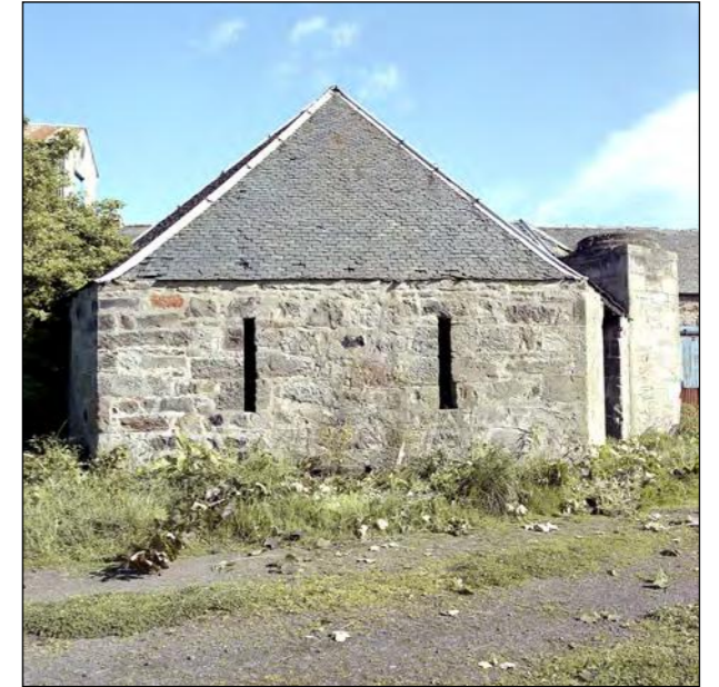
Plate 4 - Range A, South elevation. Horse engine house and chimney base.
