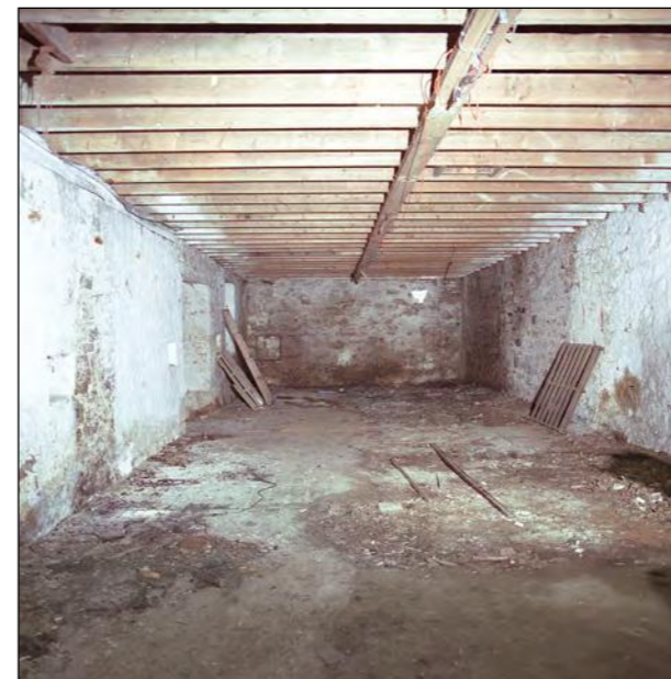
Plate 31 - Range E, Interior detail on roof timbers and floor.
