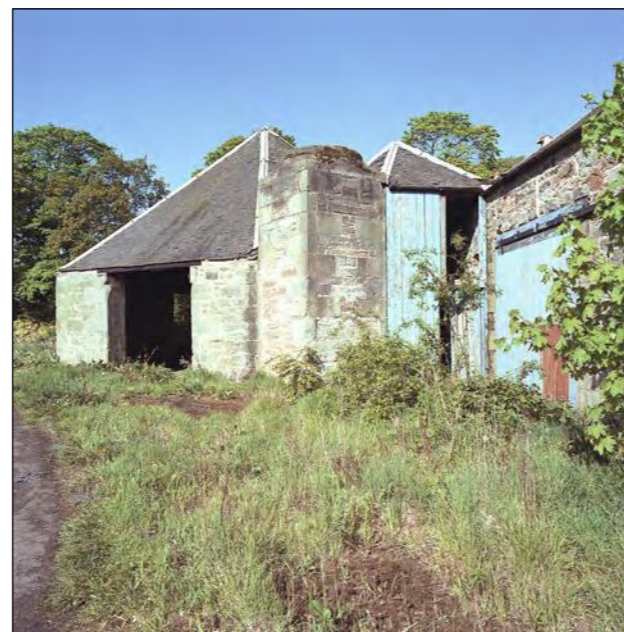
Plate 6 - Range A, East elevation showing doorway into the steam engine house.
