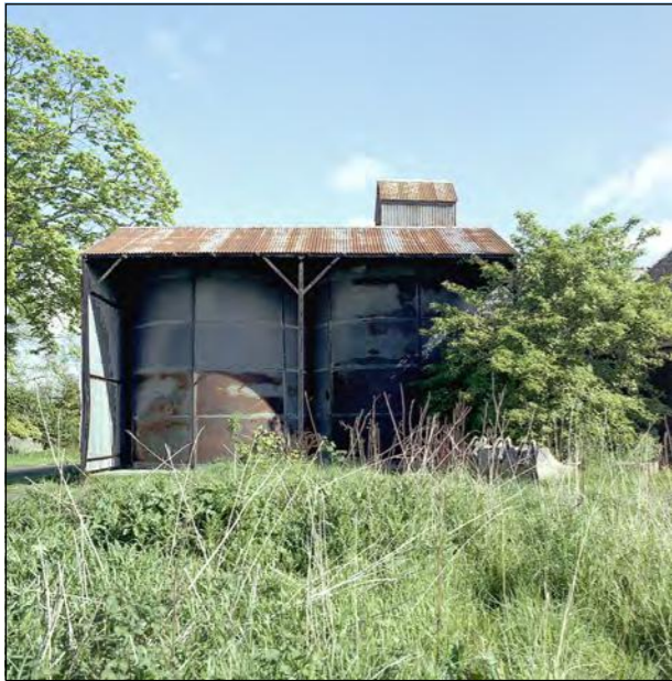
Plate 1 - Range A, South elevation. Modern grain silos.
