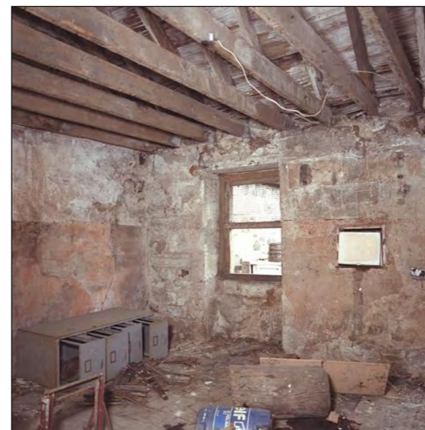
Plate 55 - Range C, Interior of stable, looking east to window.
