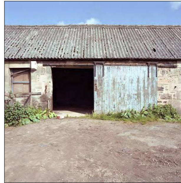
Plate 26 - Range D, South elevation with large entrance and sliding door.
