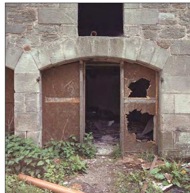
Plate 39 - Range B, West elevation, cart bay and surrounding ashlar detailing.
