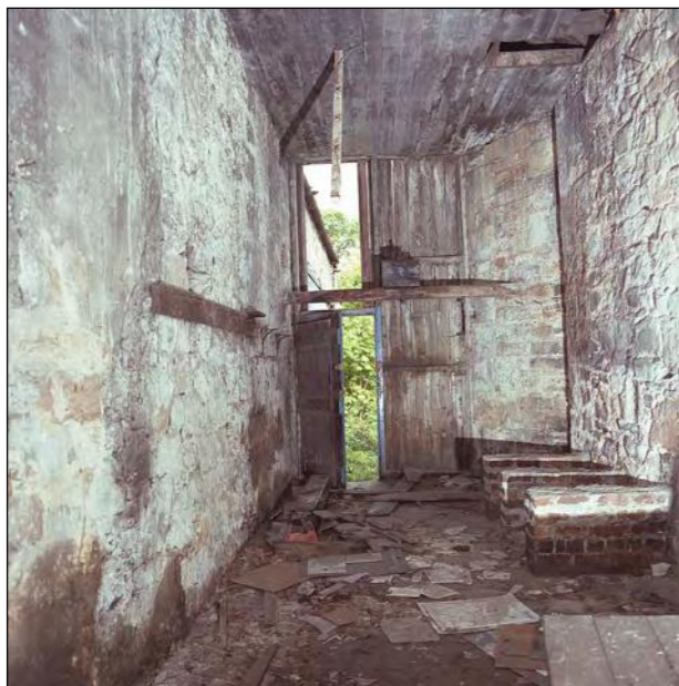
Plate 45 - Range A, Interior of the Steam Engine House, looking east.
