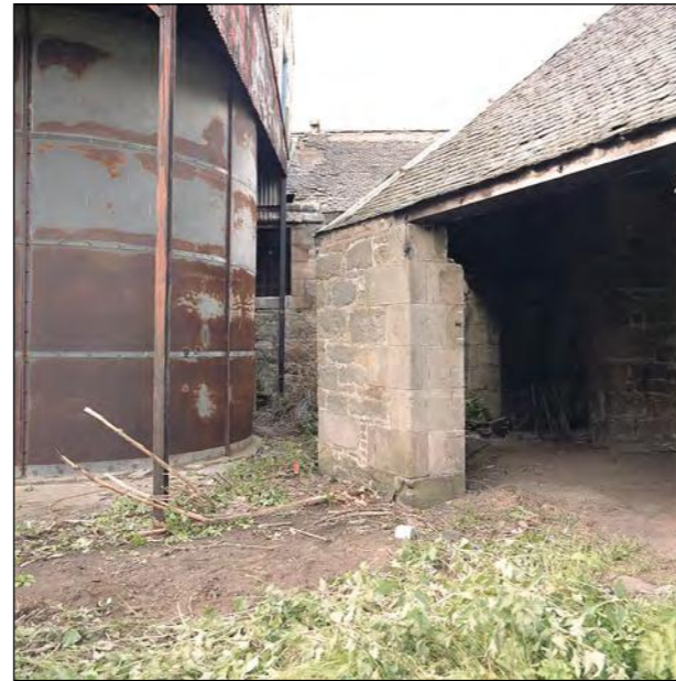
Plate 2 - Range A, South elevation. Entrance into the horse engine house.
