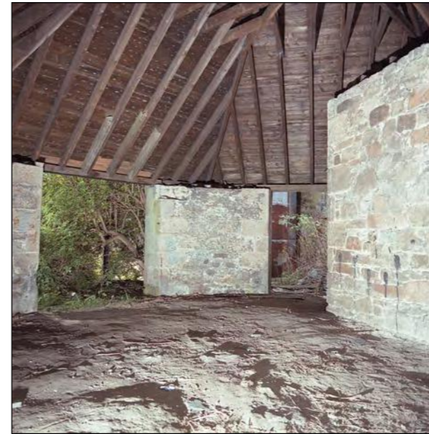
Plate 43 - Range A, Horse Engine House floor and roof, looking west.
