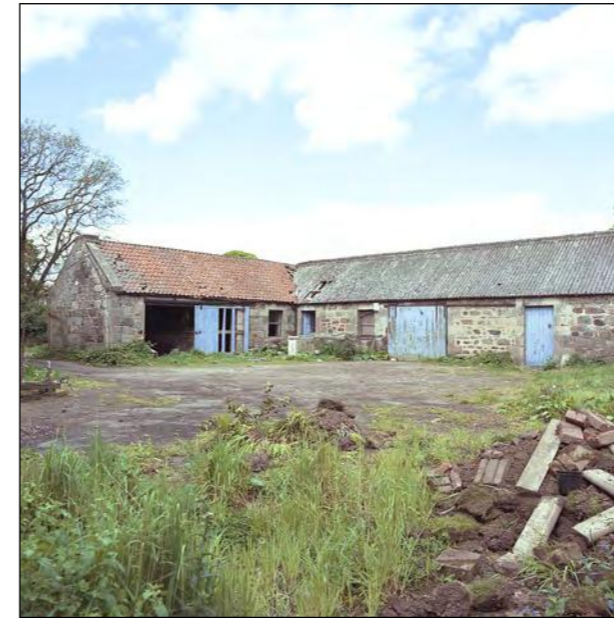
Plate 19 - Ranges C and D looking north-west and courtyard area.
