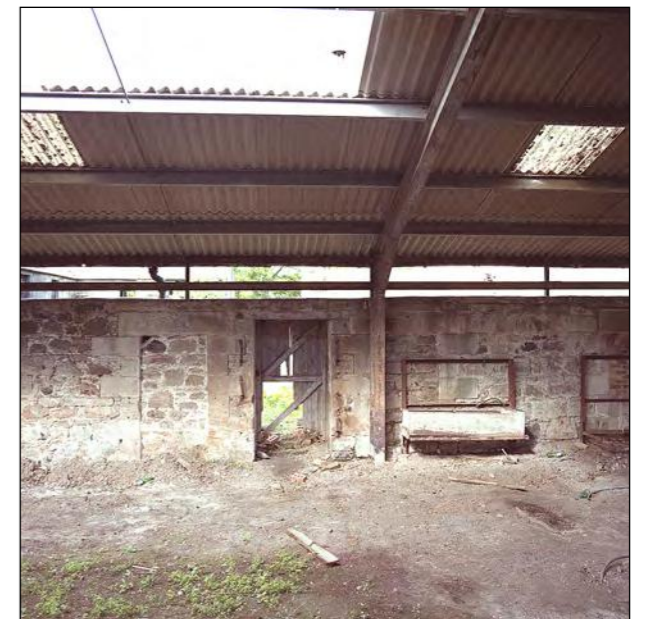
Plate 48 - Wall F. Support wall showing blocked doors and windows.
