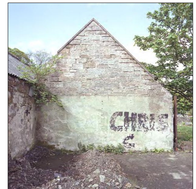
Plate 24 - Range E, East facing gable end with Range D to left of picture.
