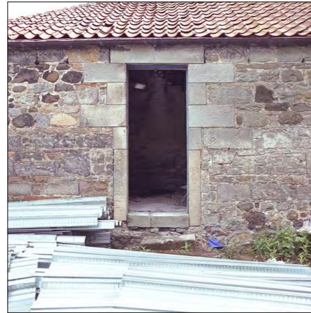
Plate 34 - Range C, West elevation entrance to storeroom.
