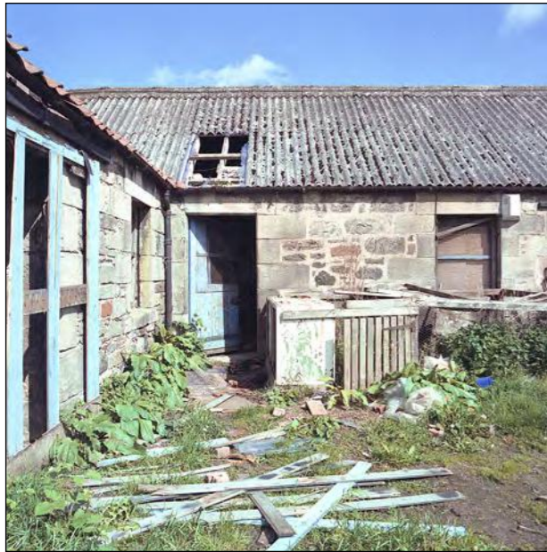
Plate 25 - Range D, South elevation and entrance to stable with blocked window.
