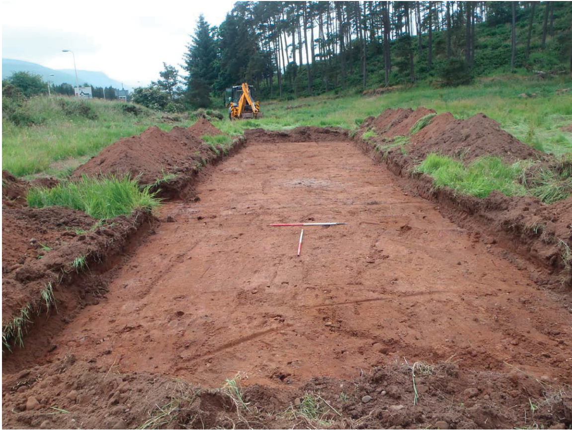
Fig. 7 - Trench 21, looking South
