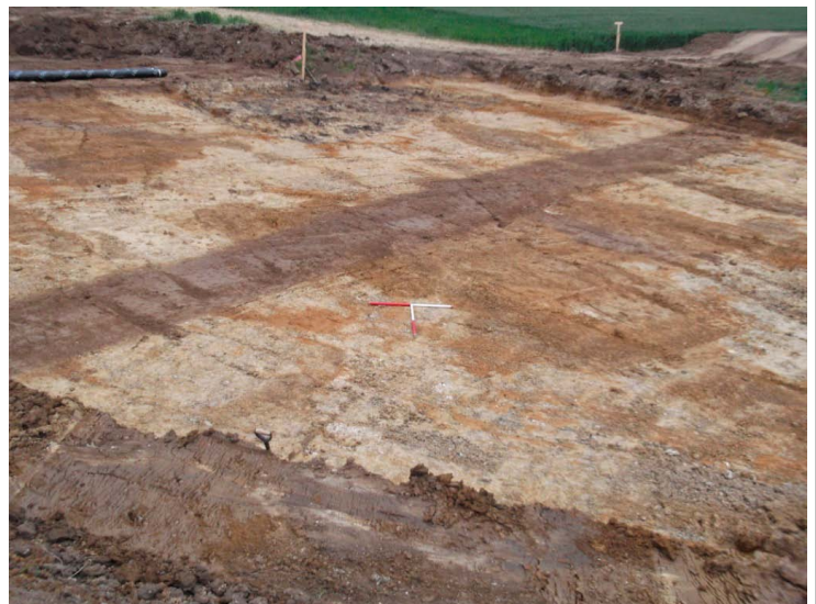
Fig. 5 - North-east-facing shot of Turbine Base 1 following topsoil removal
