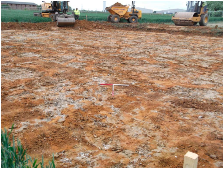
Fig. 2 - North-west-facing shot of Turbine Base 2 following topsoil removal
