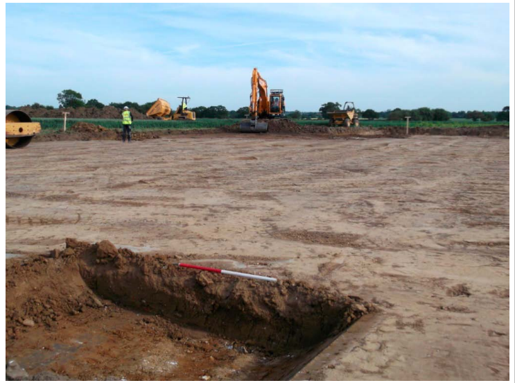
Fig. 3 - South-east-facing shot of Crane Pad 1 following topsoil strip removal
