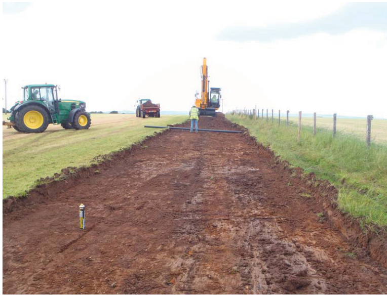
Fig. 2 - General shot looking west of topsoil strip of access track
