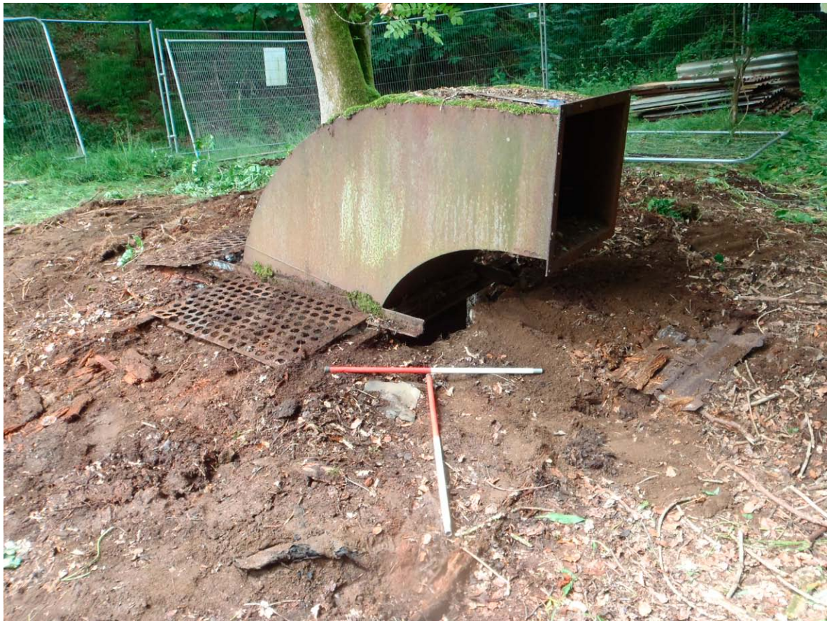
Fig. 2 - Air shaft prior to excavation
