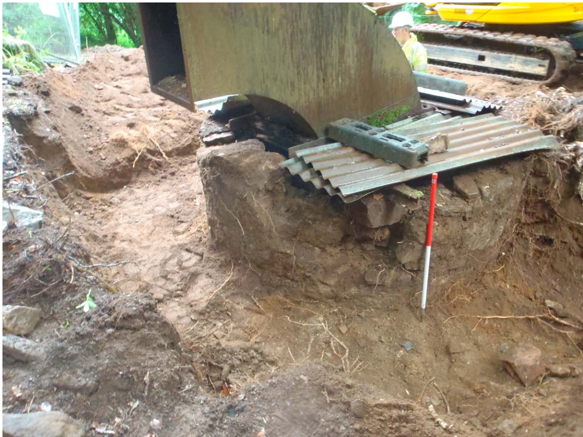
Fig. 5 - Air shaft post excavation
