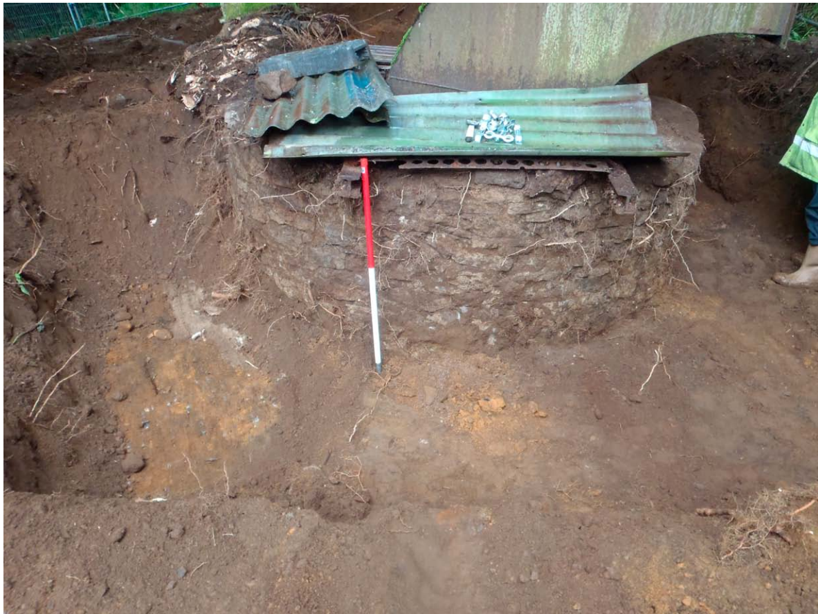
Fig. 4 - Air shaft post excavation
