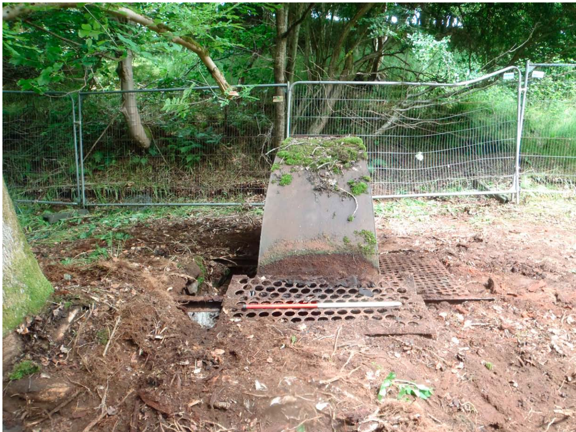
Fig. 3 - Air shaft prior to excavation
