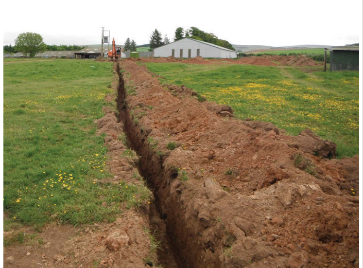
Fig. 3 - Excavated cable trench across field
