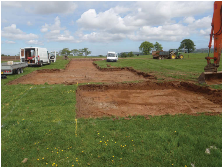
Fig. 2 - Turbine base and crane pad stripped of topsoil from SW
