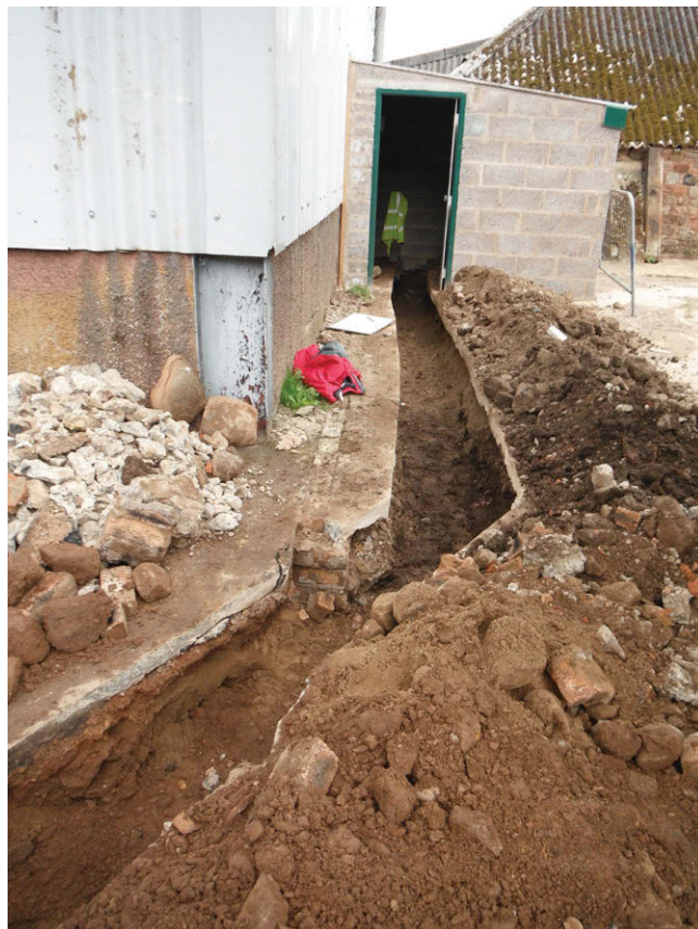
Fig. 4 - Excavated cable trench across farm yard
