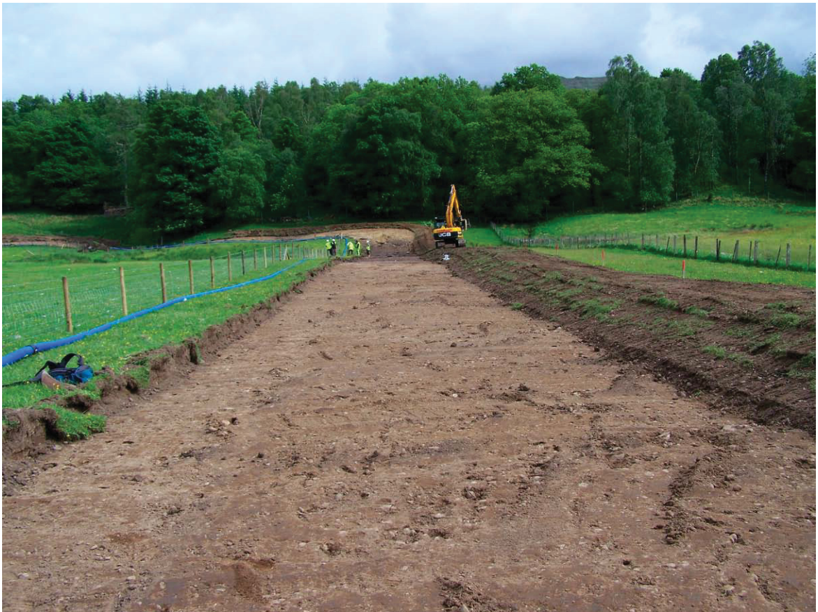
Fig. 3 - View of stripped pipeline wayleave from NE
