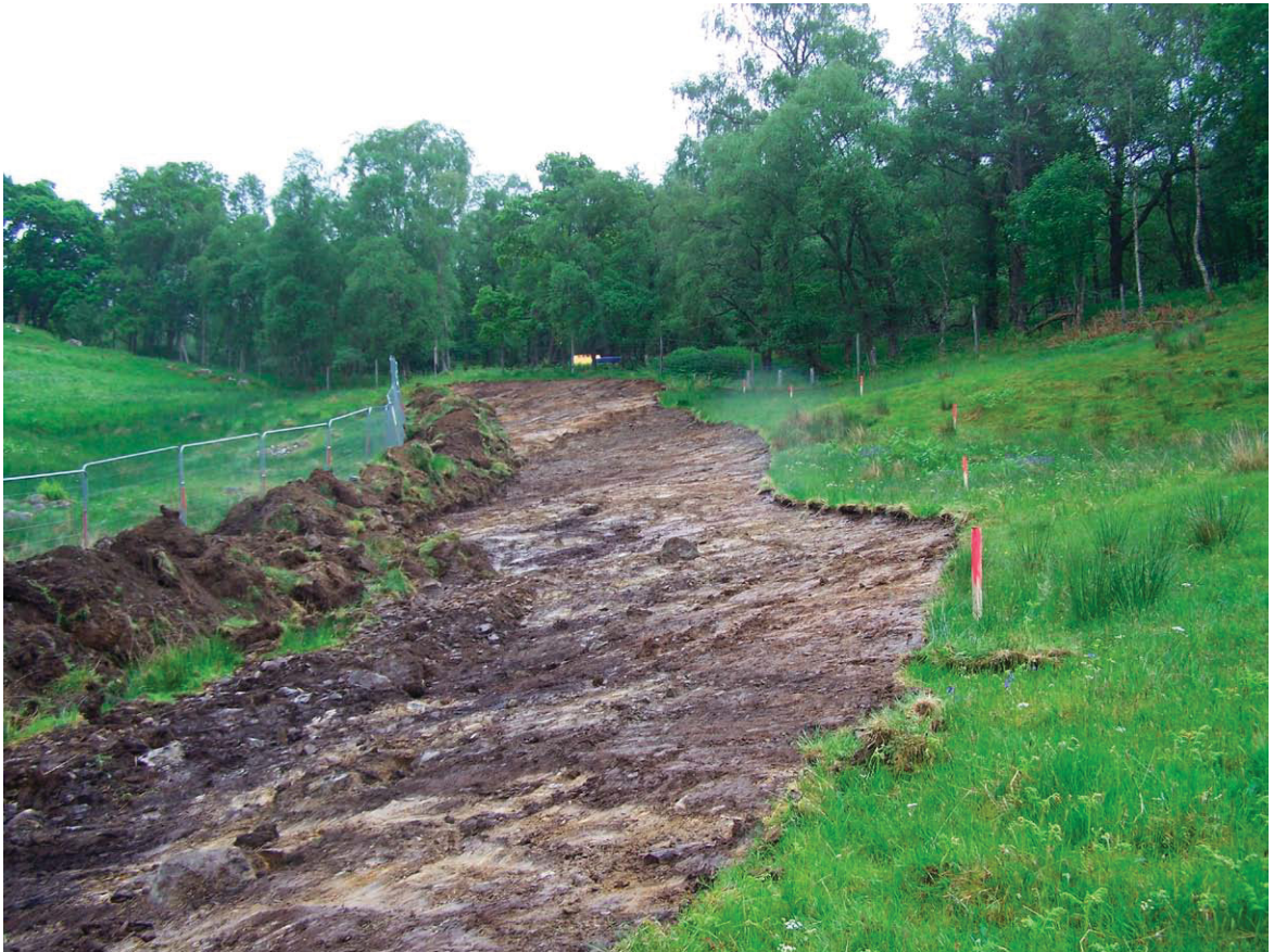
Fig. 2 - View of stripped pipeline wayleave from NW
