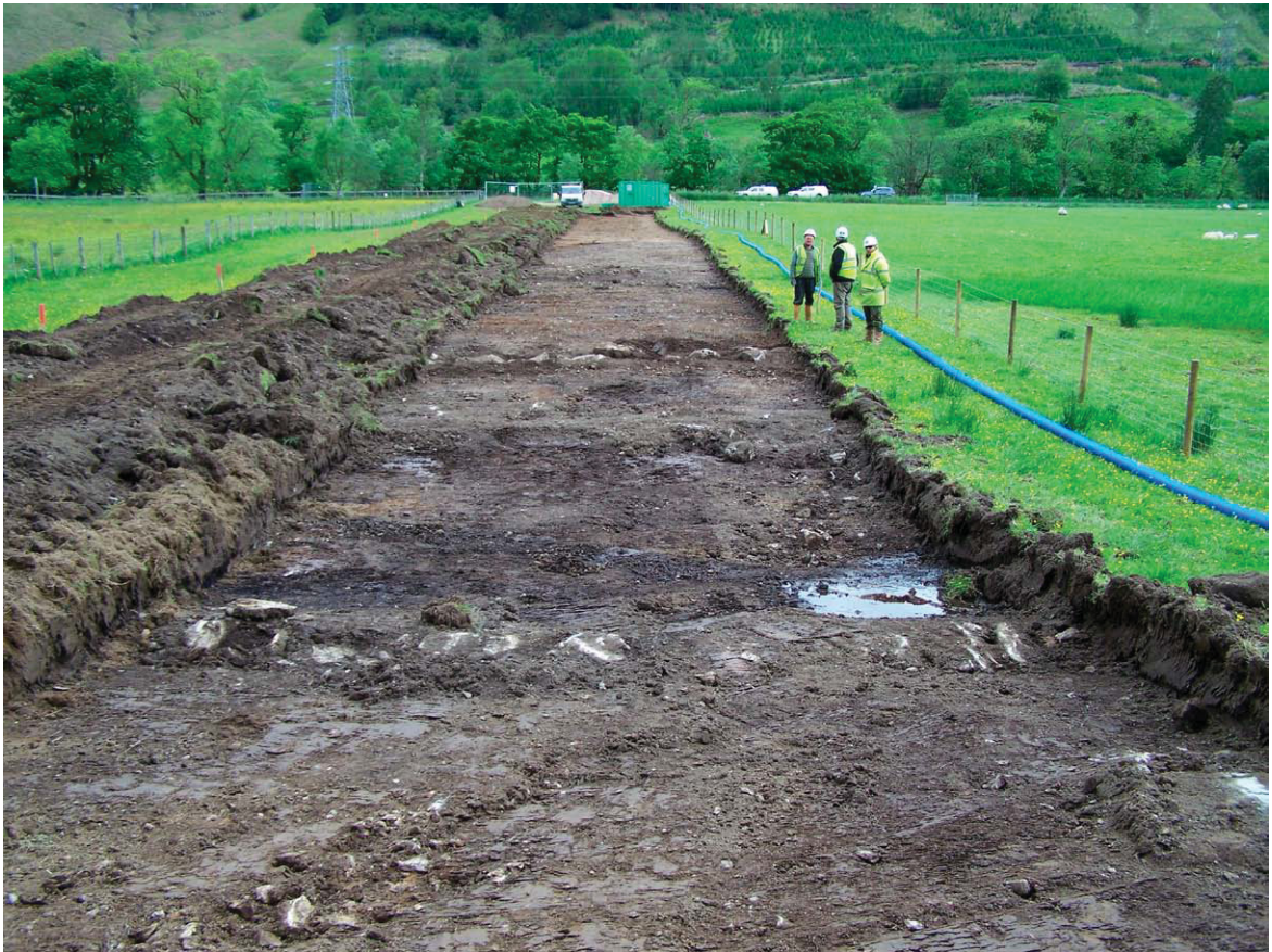
Fig. 4 - View of stripped pipeline wayleave from SE
