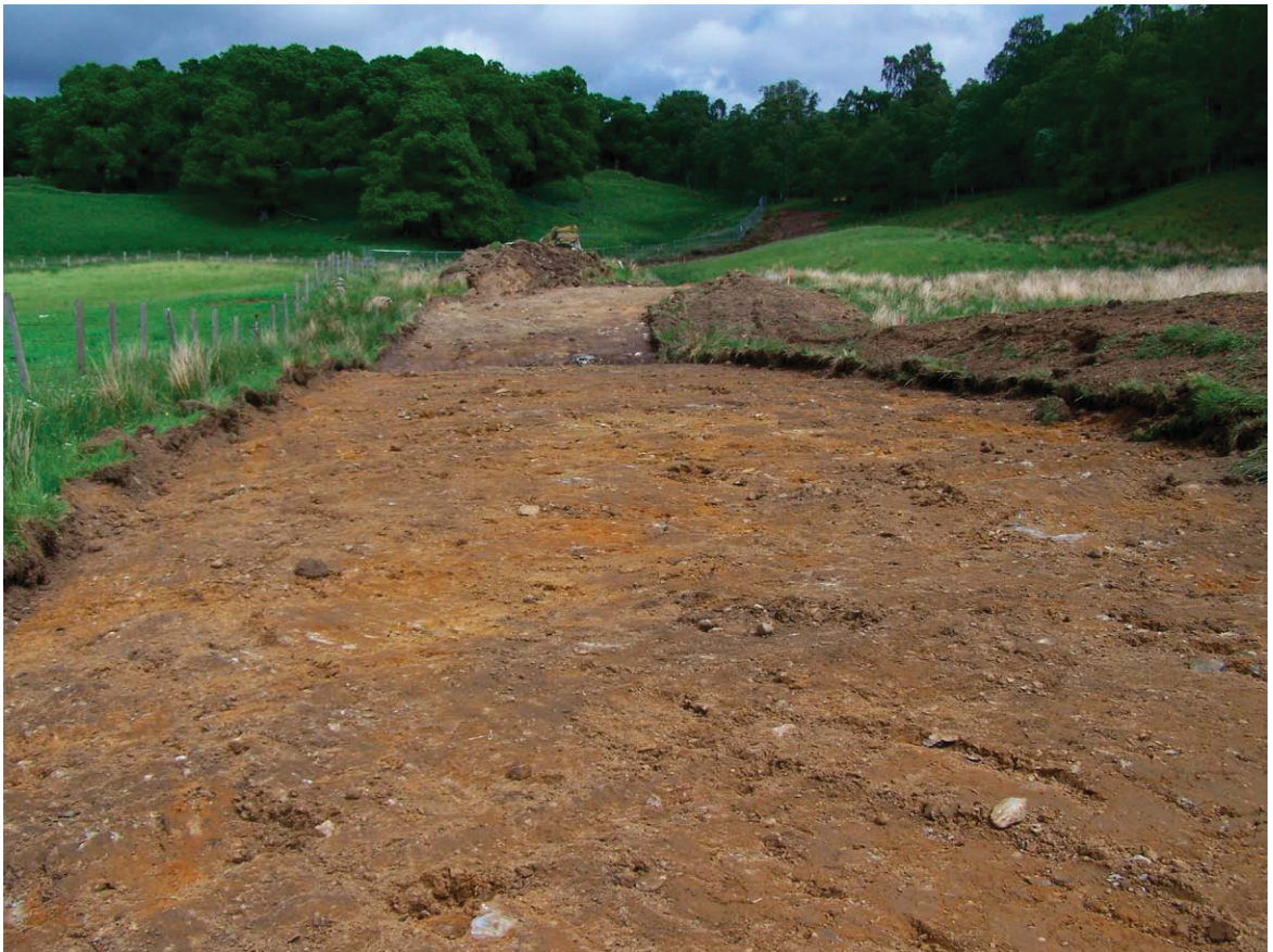
Fig. 3 - View of stripped pipeline wayleave from SW
