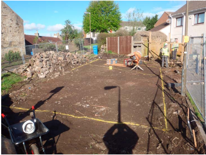
Fig. 2 - Site stripped of surface turf
