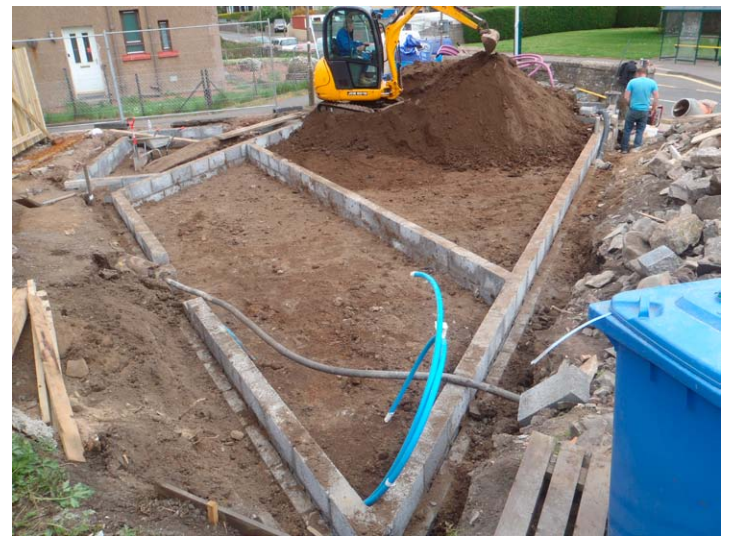
Fig 5. - General view of site fully excavated
