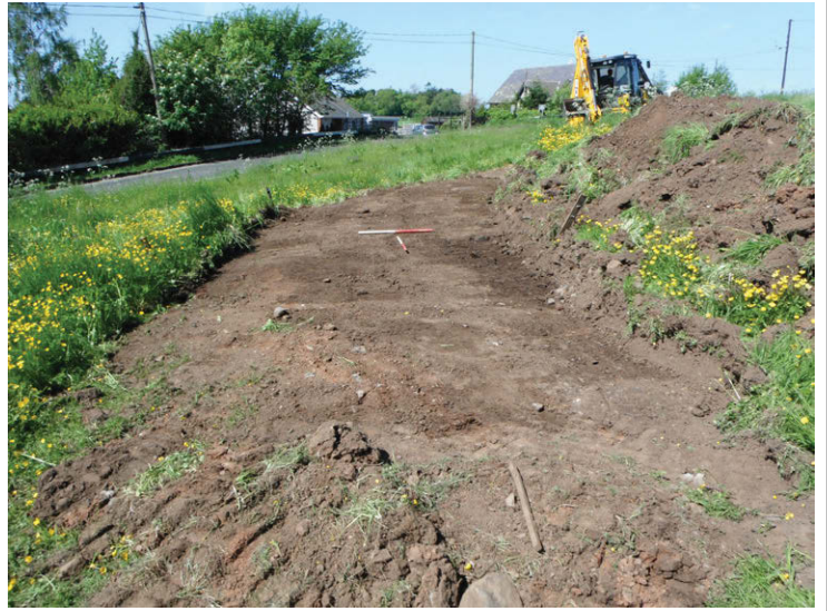
Fig. 3 - Access road 2, from E
