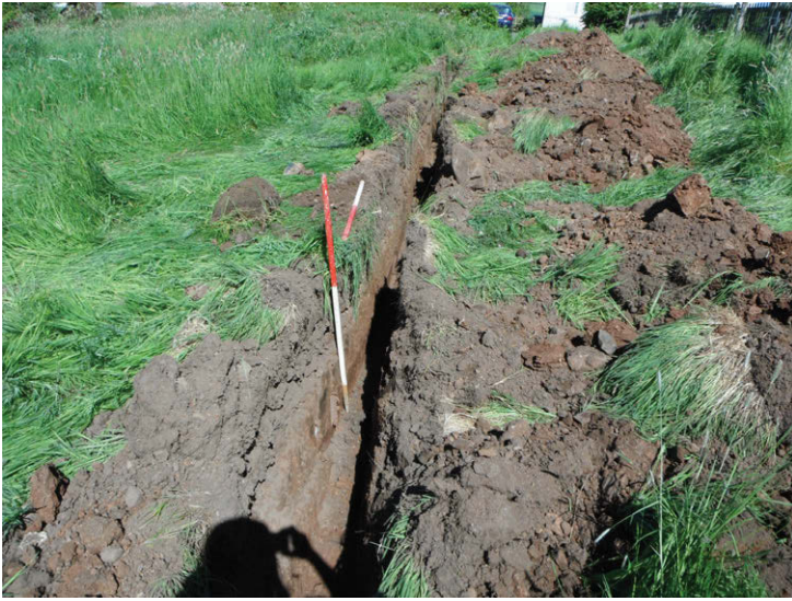
Fig. 2 - Water pipe excavated, from SE
