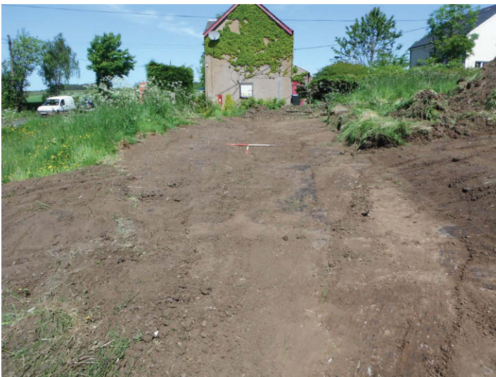
Fig. 5 - Access road 1, from NW
