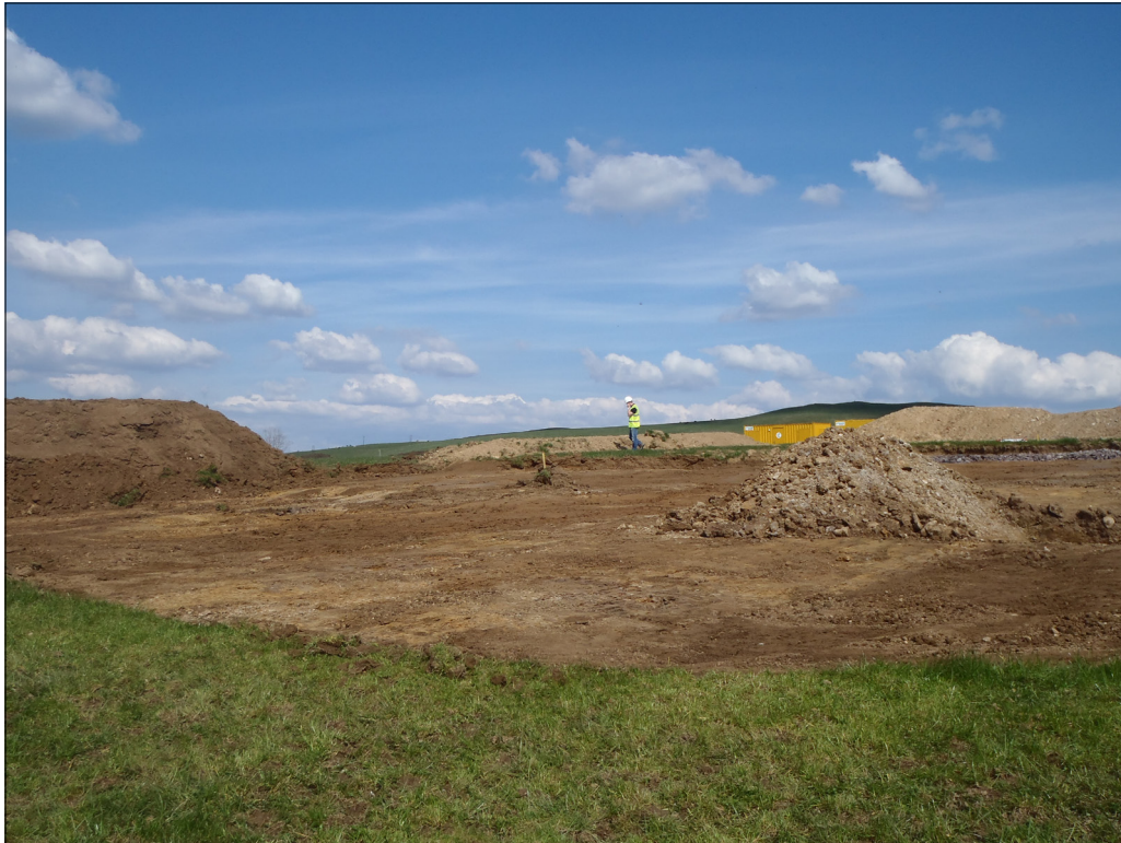
Fig. 6. - General view of crane pad and turbine base
