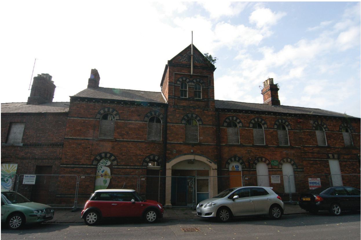
Plate 6 - Centre of the north-facing elevation showing the drill hall (Building 2)
