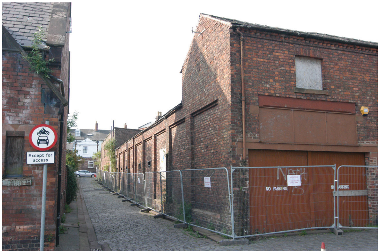
Plate 8 - East gable and walls of the Swift Mews courtyard (Building 4)
