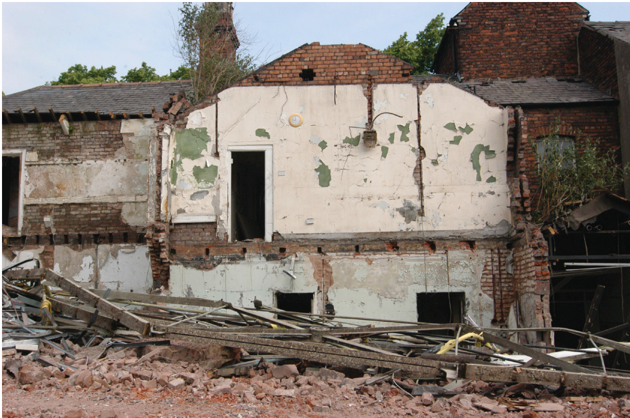
Plate 10 - South-facing elevation showing the remains of a demolished (rear blocks of Building 2)
