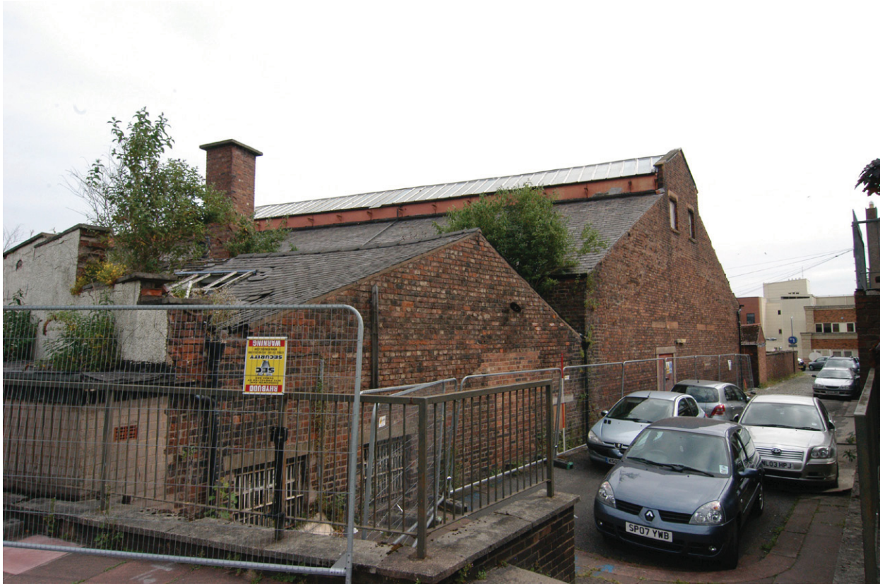
Plate 17 - South-facing gable of Building 7 adjoining Building 5
