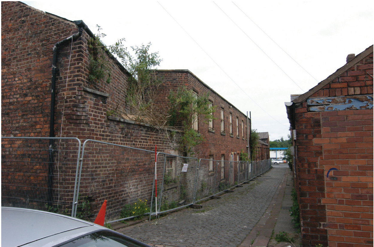
Plate 16 - East-facing elevation of Building 6 with barred windows and flat roof
