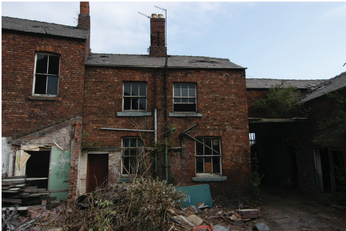
Plate 12 - South-facing elevation of the Swift Mews (Building 3)
