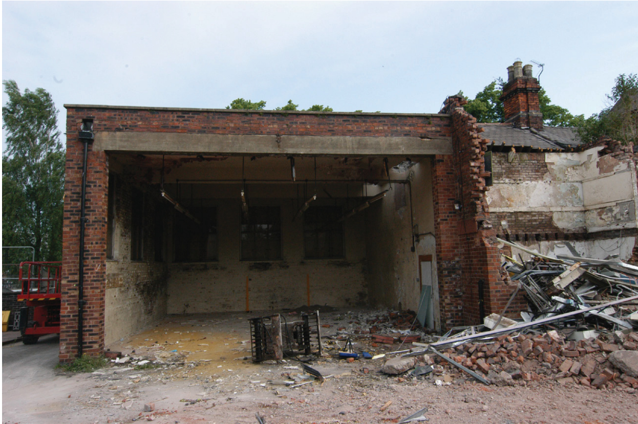
Plate 9 - South-facing elevation of the workshop/garage (Building 1)
