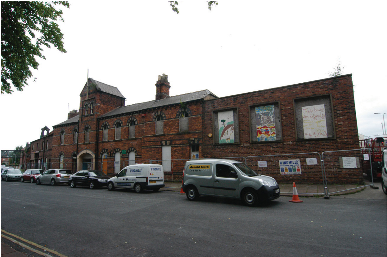
Plate 5 - West end of the north-facing elevation showing workshop (Buildings 1 and 2)
