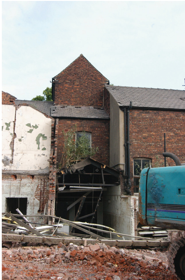
Plate 11 -South-facing elevation of Building 2, passage and adjoining structures
