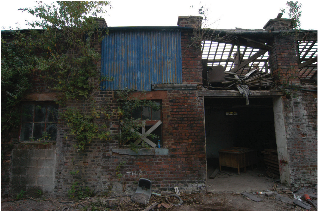
Plate 13 - One of the mews courtyard buildings with king-post roof truss exposed (Building 4)
