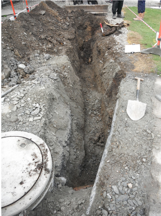
Fig. 5 Pipeline excavated to a length of 4m
