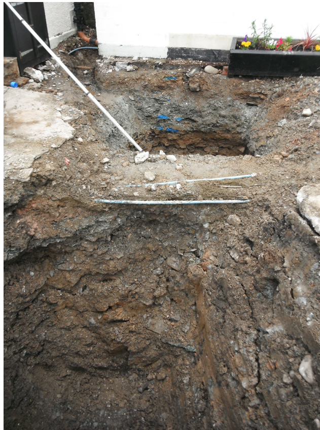
Fig. 4 Trench 1 and 2 fully excavated
