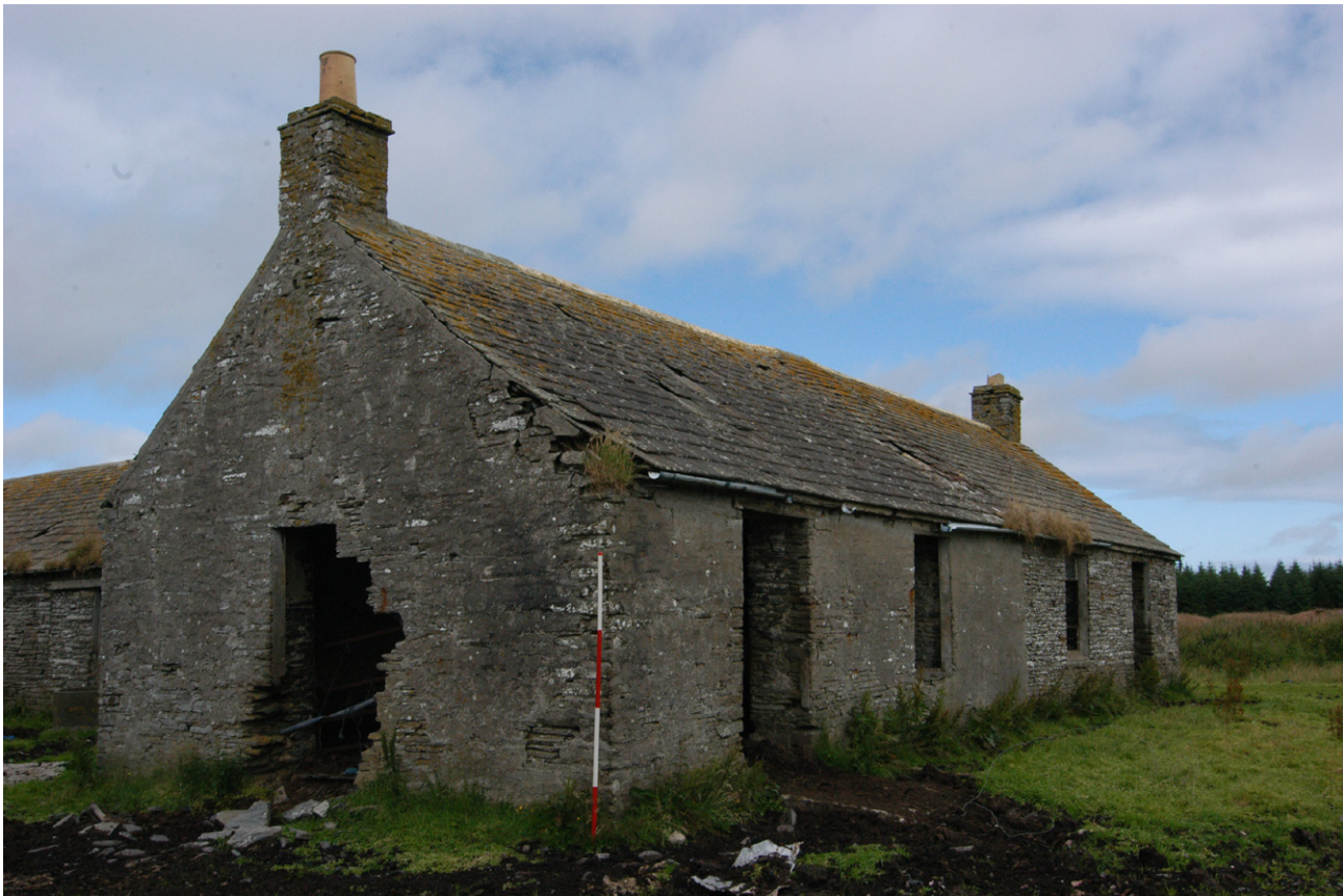
Plate 2 - General view of the gable and collapsed central window
