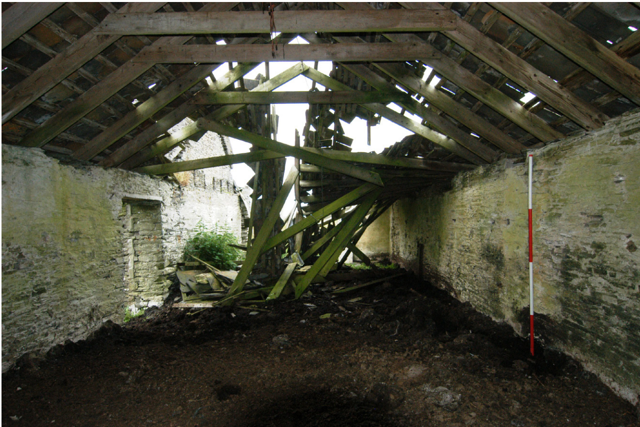
Plate 22 - Interior north-west end of Unit 6 showing collapsed roof
