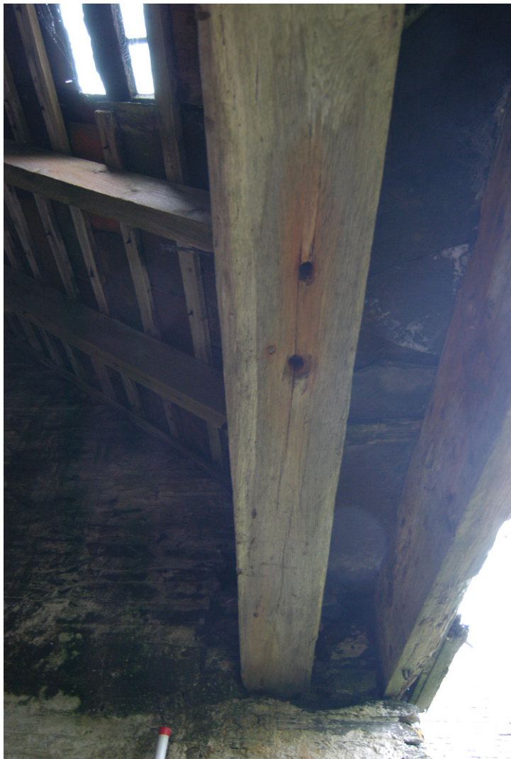
Plate 19 - Detailed shot of the underside of the possible ship's timber with drill holes
