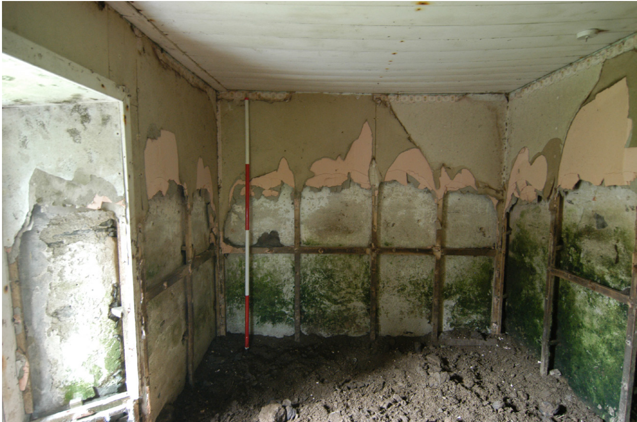
Plate 15 - Interior of Unit 3 showing wall cladding
