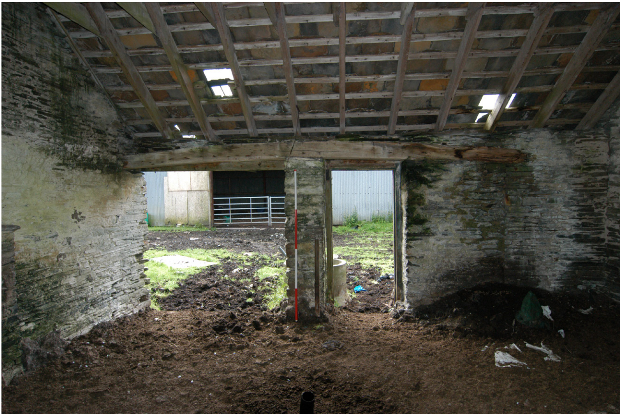
Plate 18 - Interior view of the door openings in Unit 5 with a possible re-used ship's timber
