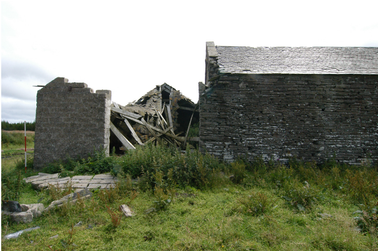
Plate 5 - Collapsed gable wall of the byre (Unit 60), north-west-facing elevation
