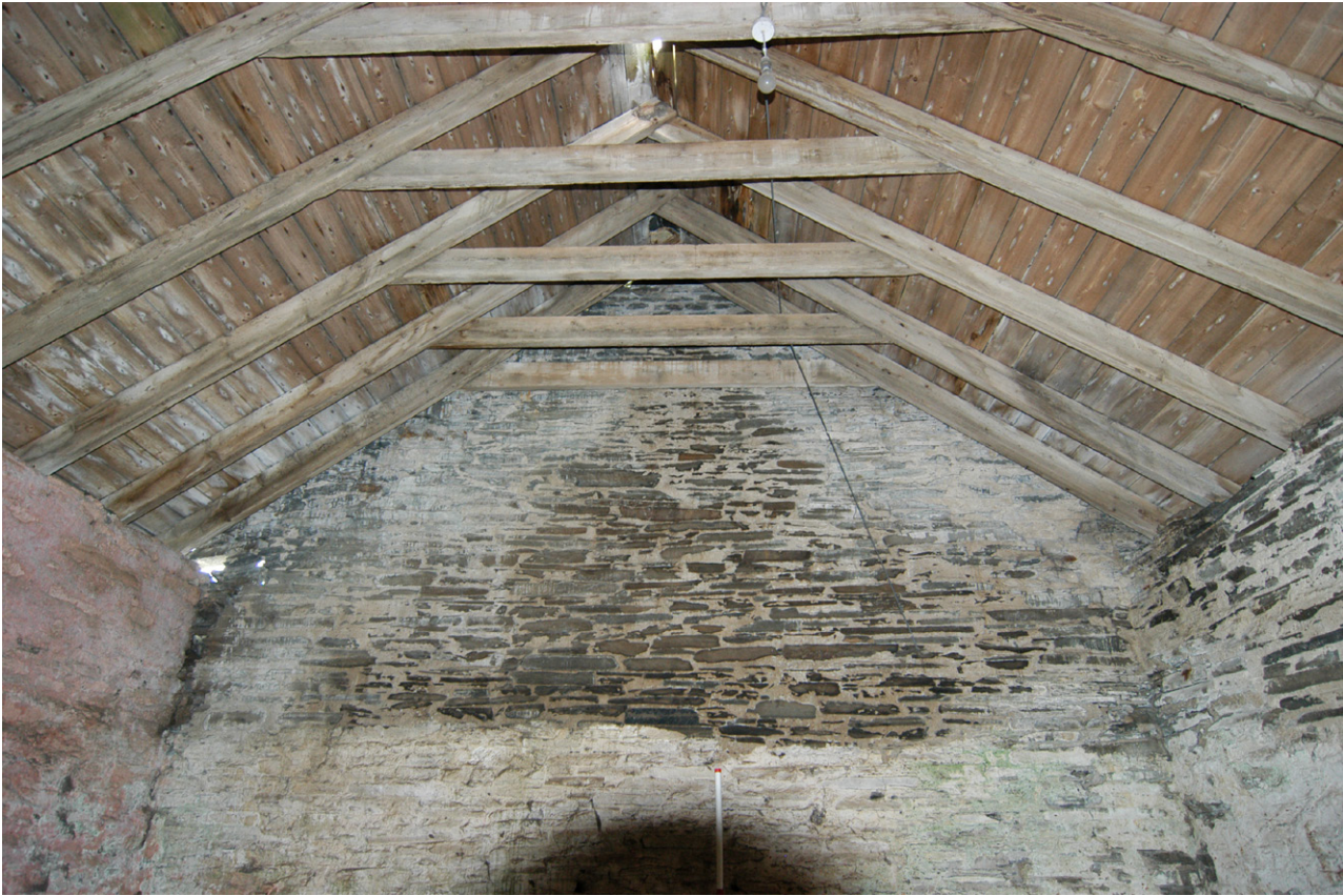
Plate 24 - Interior south-west facing gable of the threshing barn showing wall heightening
