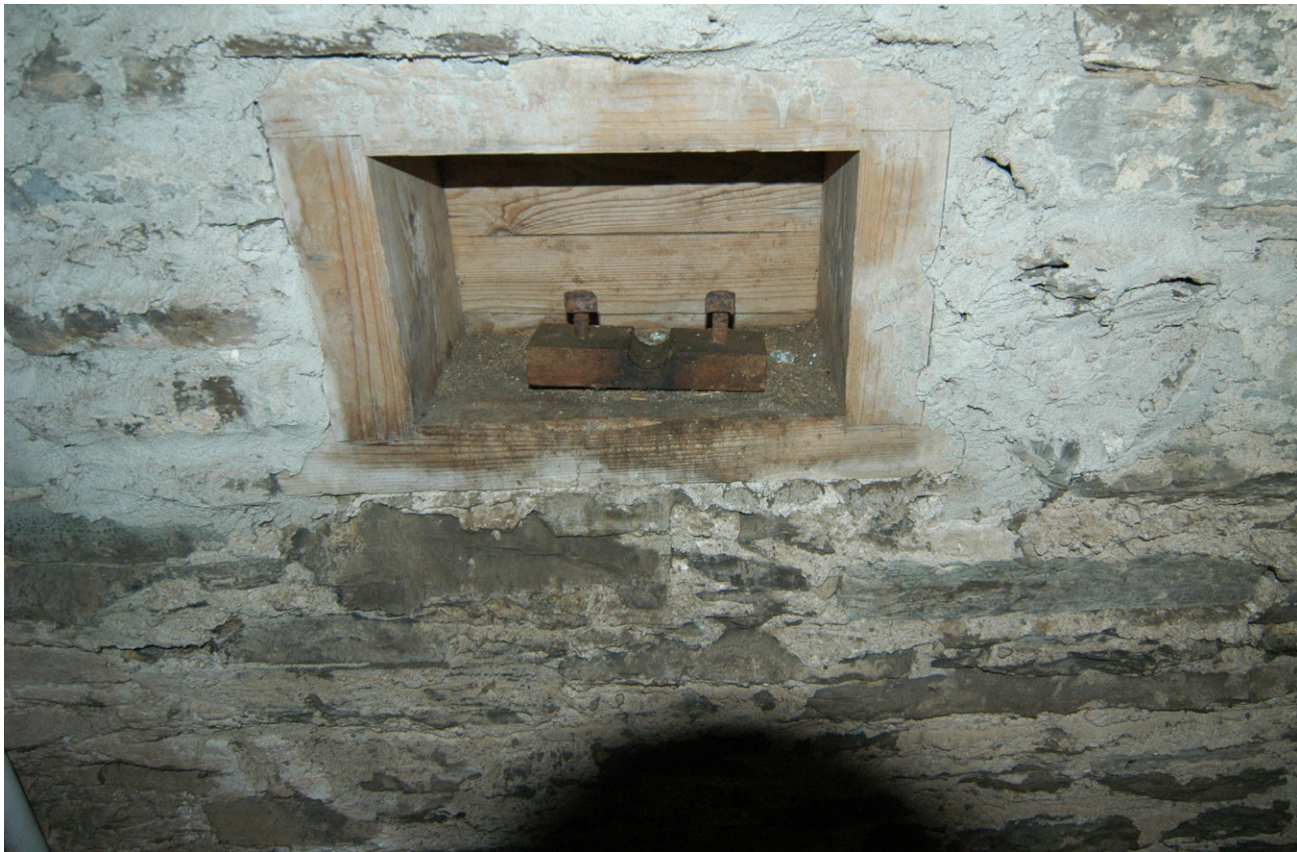
Plate 26 - A bearing box at loft level
