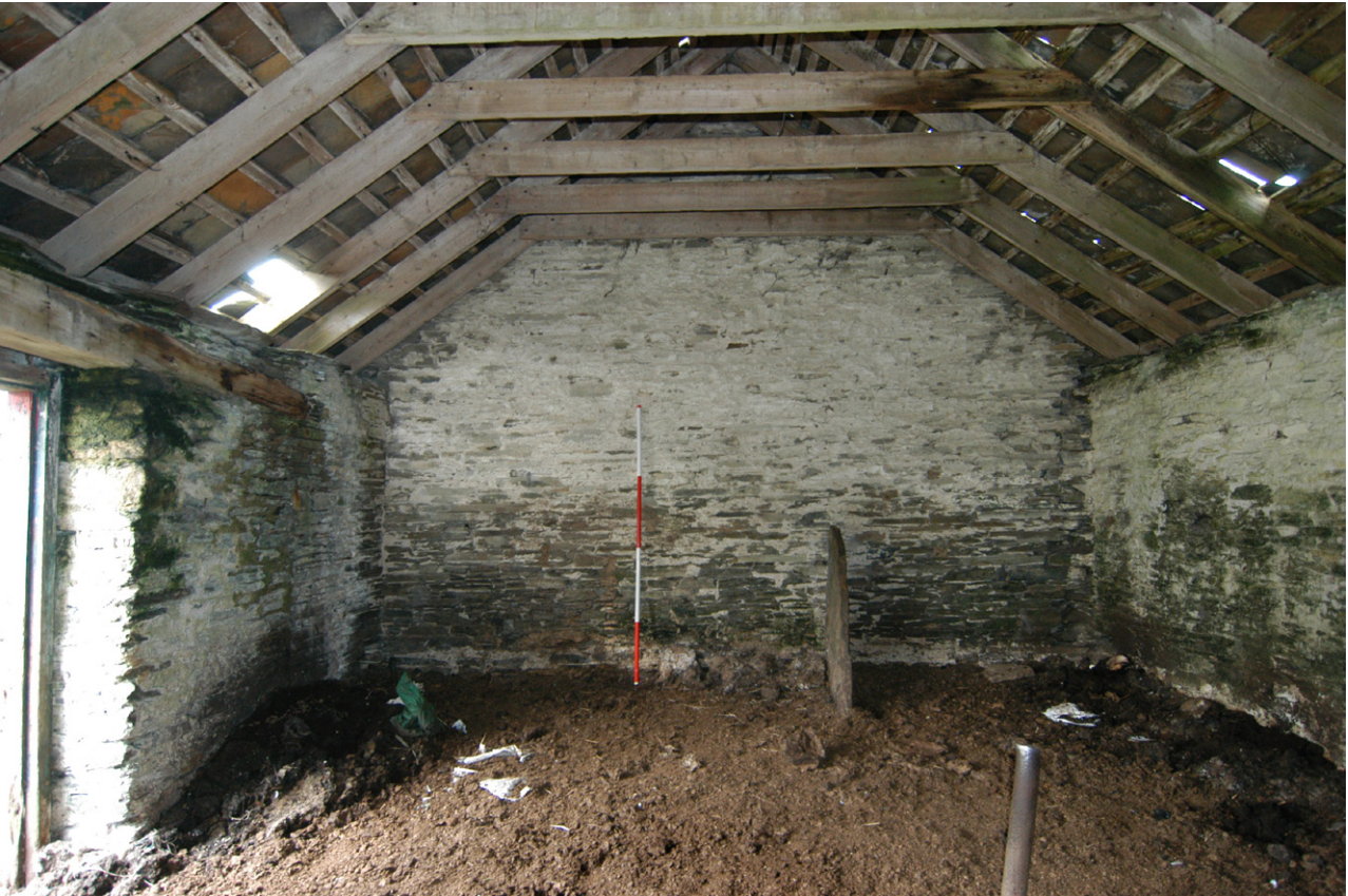
Plate 20 - Interior south-east-facing wall with a stall made from a large fireplace
