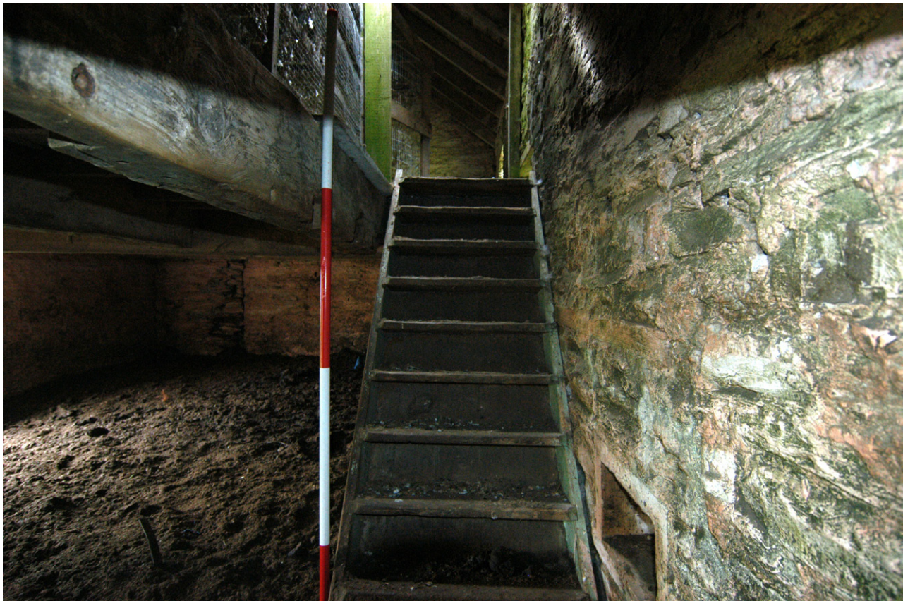
Plate 25 - Loft staircase, with a bearing box on the adjacent wall heightening
