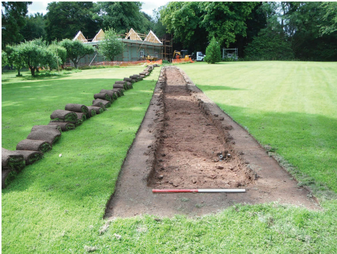
Fig. 3 View of soakaway trench post-excavation
