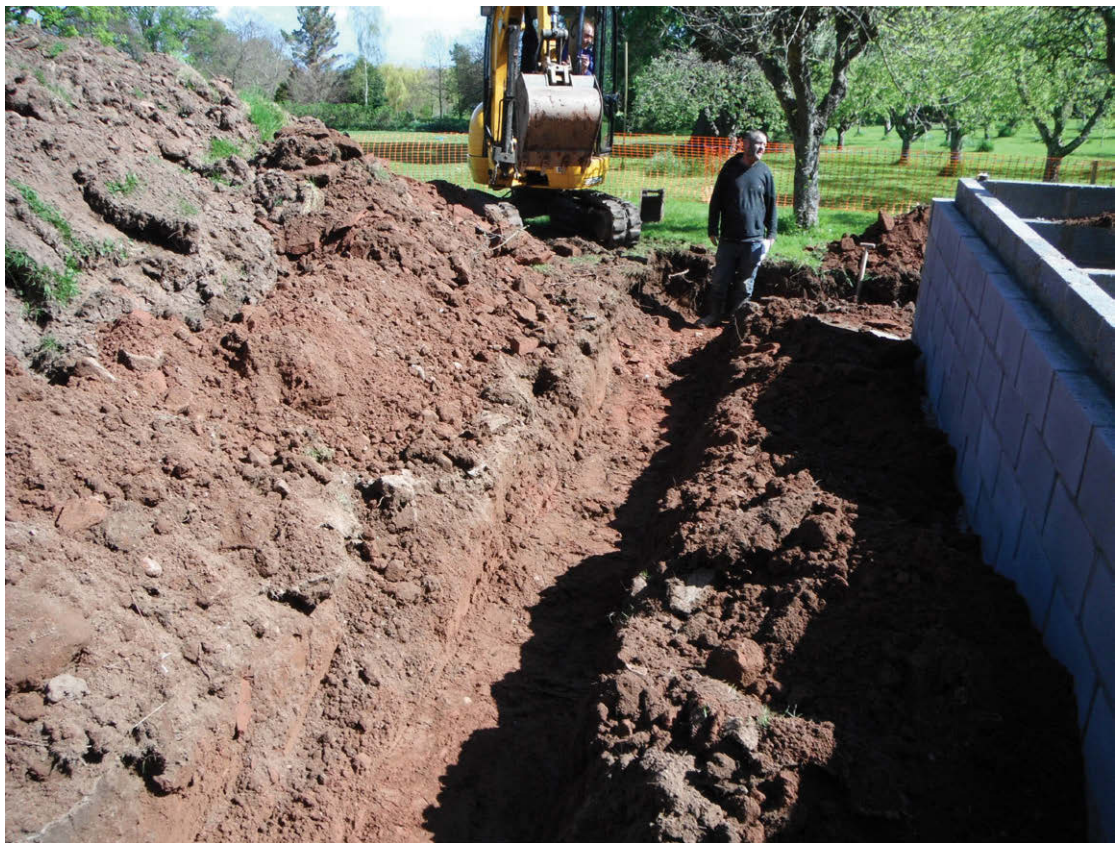
Fig. 2 View of drainage trench post-excavation
