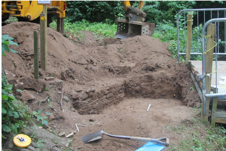
Fig. 2 - Western Bridge Abutment, post-ex
