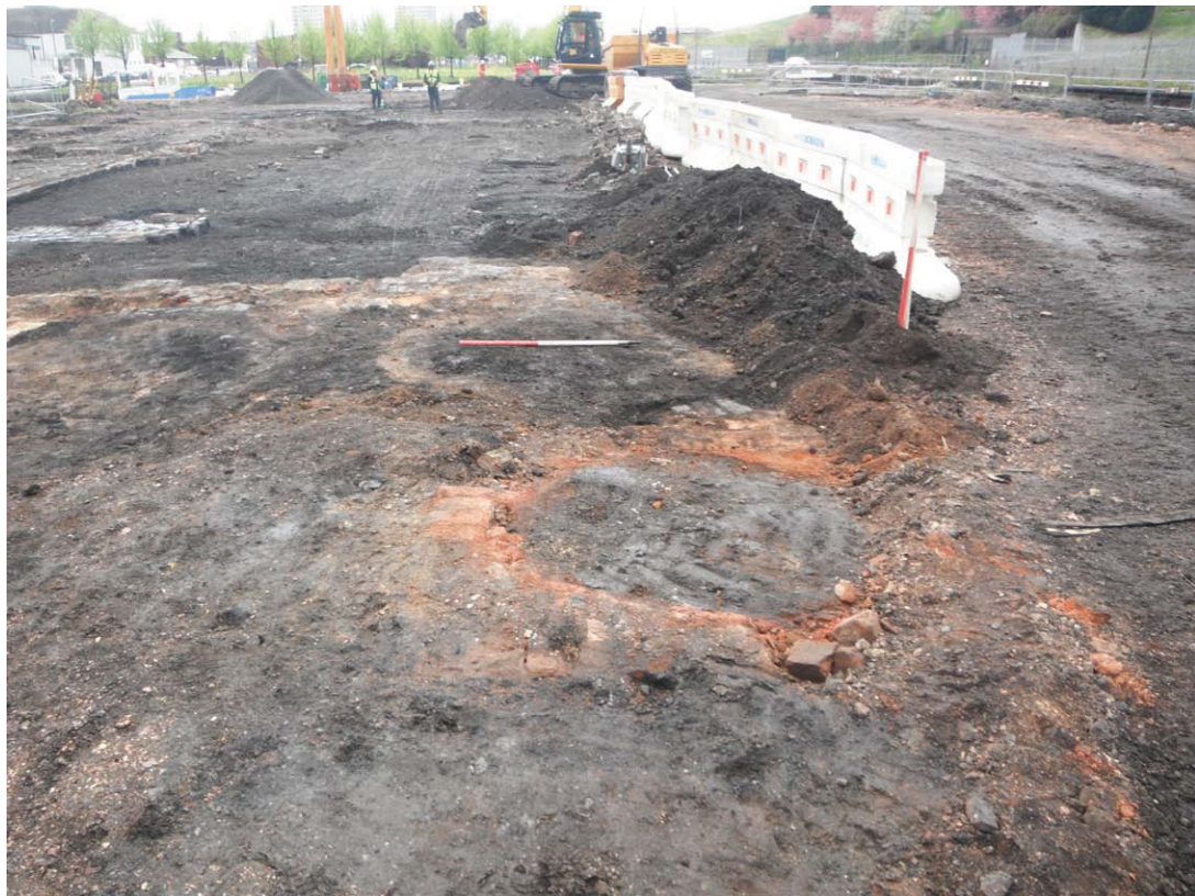
Fig. 21 - Coke oven 3 and chimney 137 in foreground
