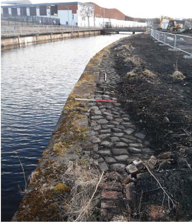
Fig. 9 - Cobbles 028 along wharf edge
