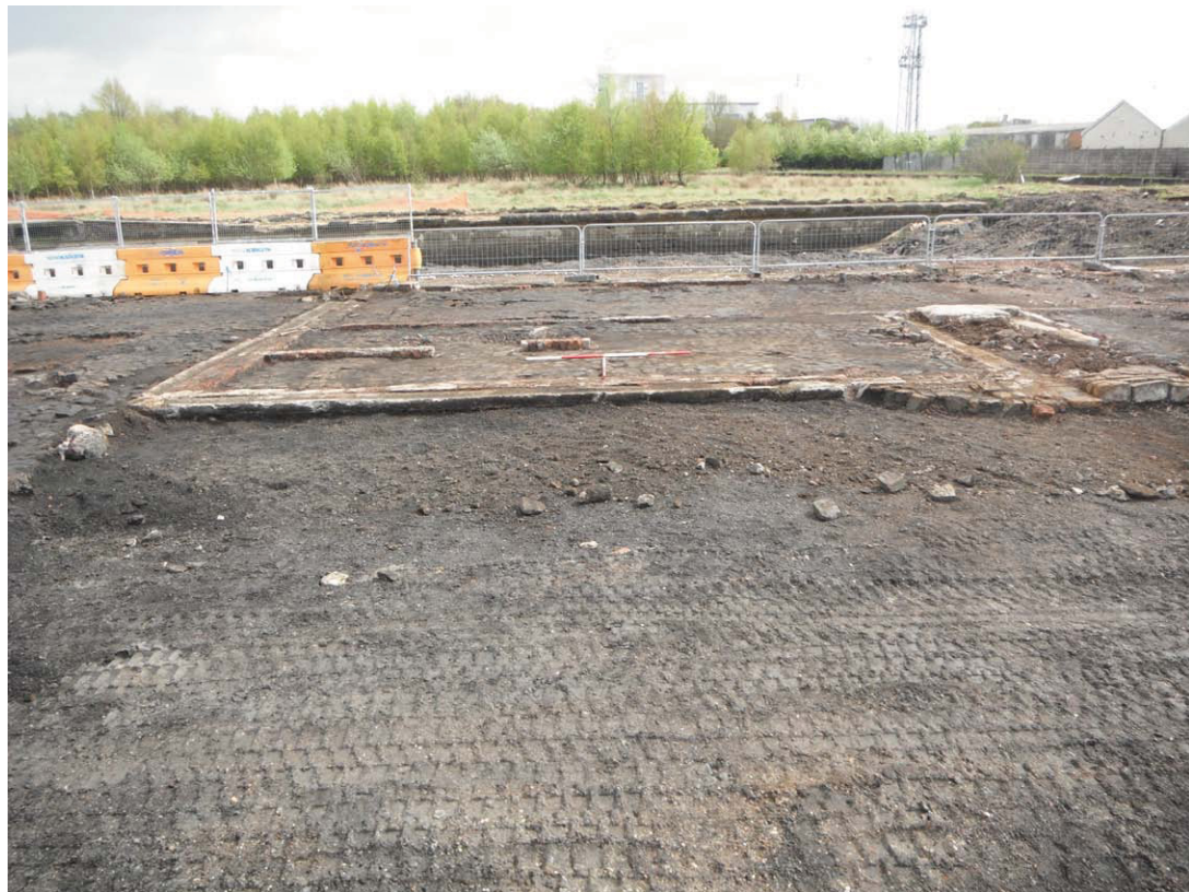
Fig. 13 - General view of building 1
