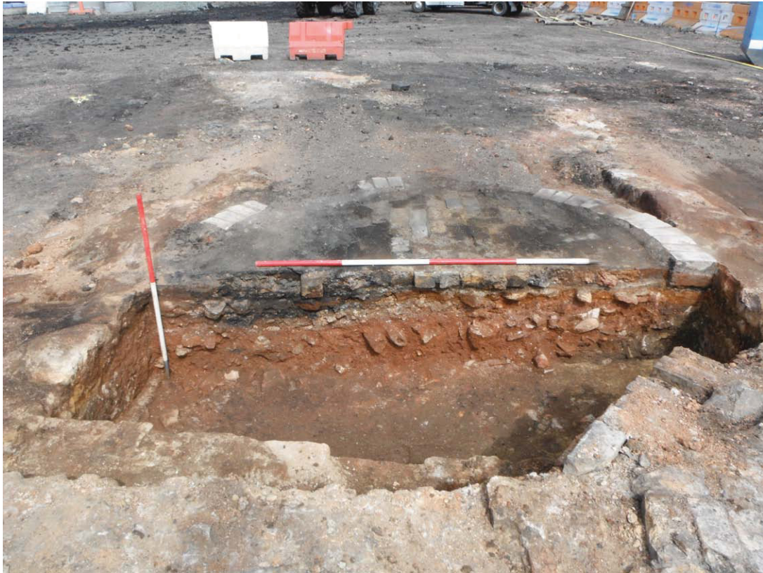
Fig. 18 - Coke oven 1 half-sectioned
