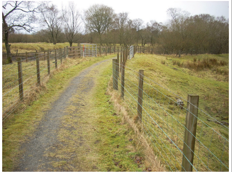
Fig. 10 - Site 10, public footpath on top of embankment, from NE
