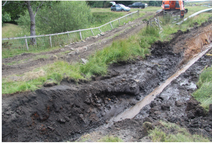
Fig. 14 - SW-facing section of canal basin with mineral embankment in foreground
