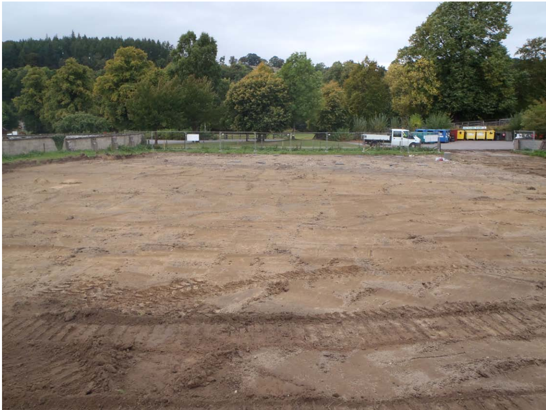
Fig 3. - View of stripped area
