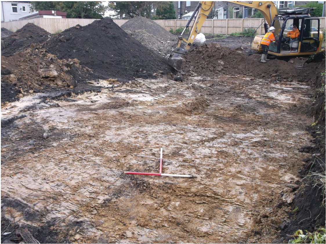
Plate. 1 - Working shot of topsoil removal at south of site
