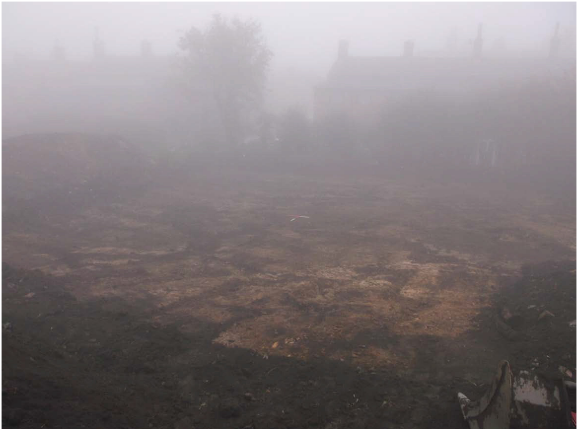
Plate. 2 - South-west-facing shot of the middle of site following topsoil removal
