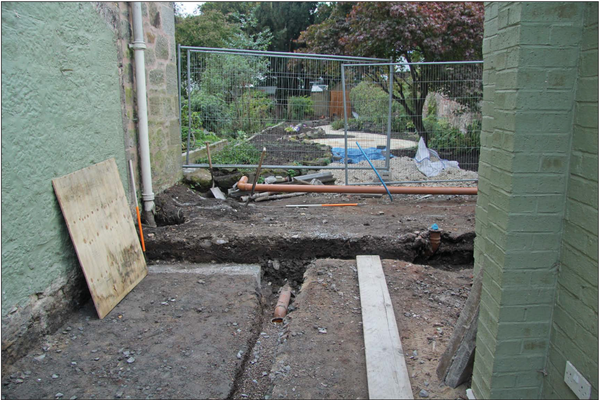
Plate 3 – Drainage and foundation trenches
