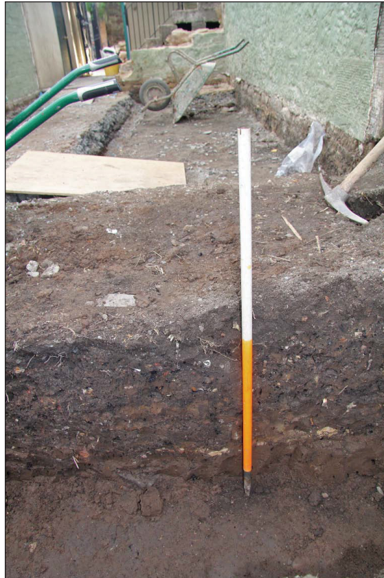
Plate 4 – Section of foundation trench
