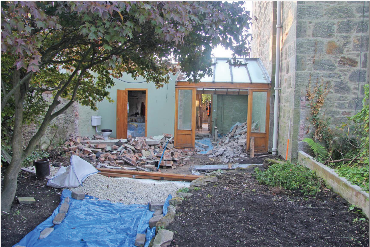
Plate 1 – General development area mid demolition
