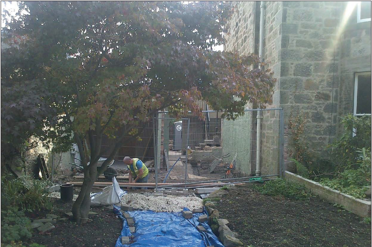
Plate 2 – General development area post demolition
