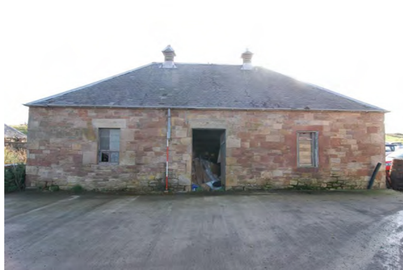
Plate 2: Building 1, north-west facing (front) elevation
