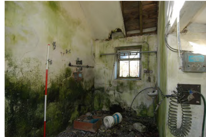
Plate 9: Building 2, Unit 2/2 wash room room
