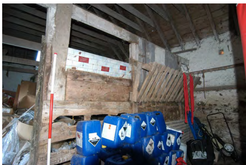
Plate 4: Building 1, interior timber stalling at south-west end
