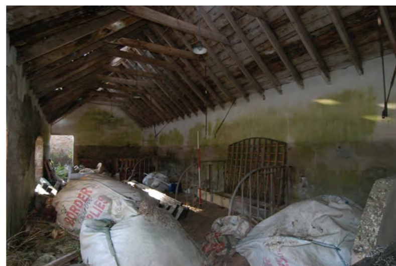
Plate 14: Building 3, Unit 3/1 interior
