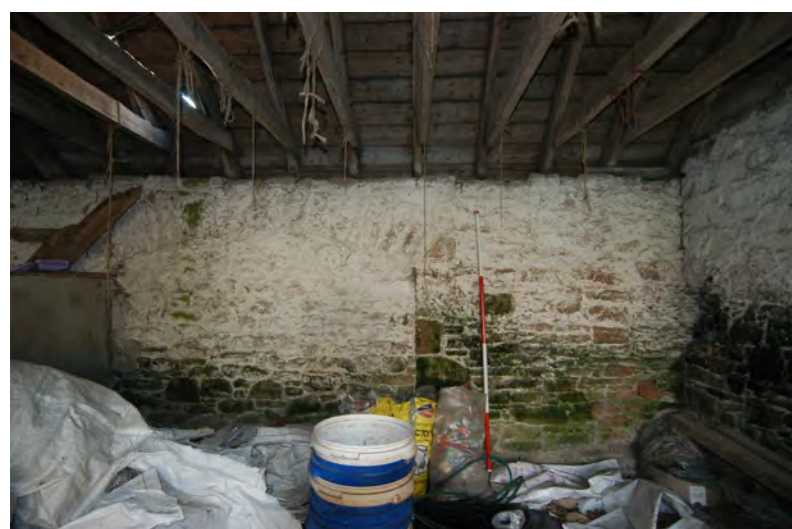
Plate 16: Building 3, Unit 3/4 interior showing blocked arch opening
