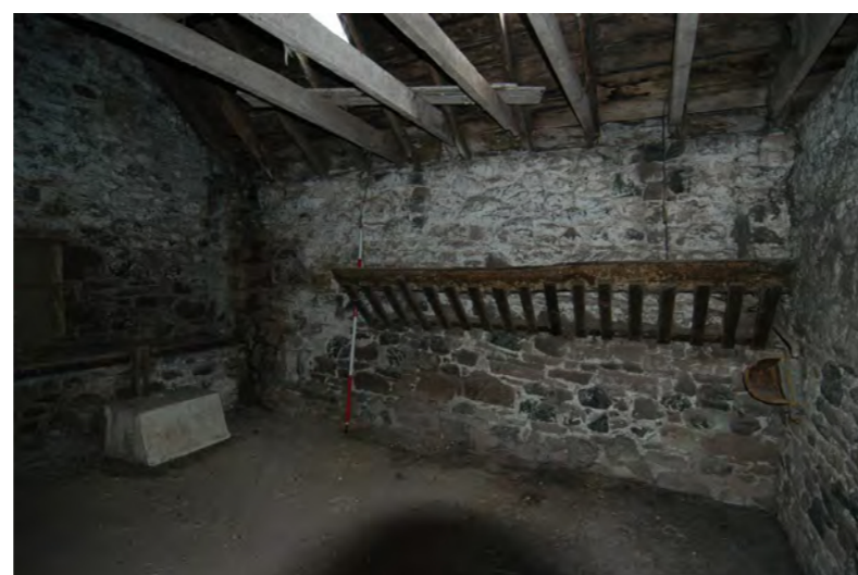
Plate 17: Building 3, Unit 3/5 interior view
