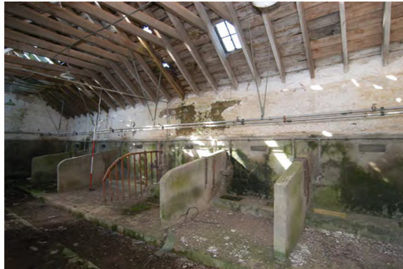
Plate 8: Unit 2/1 milking shed stalls
