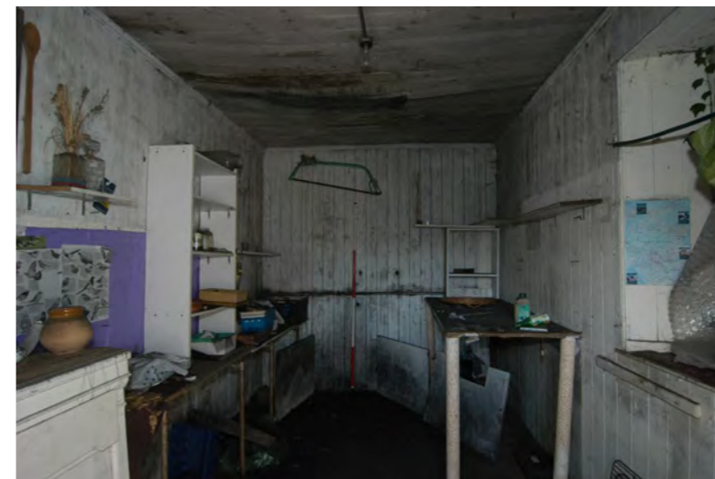
Plate 12: Building 2, Unit 2/5 workshop interior
