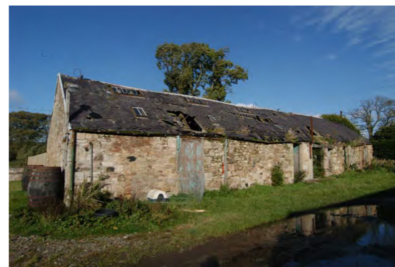
Plate 6: Building 2, south-east facing elevation
