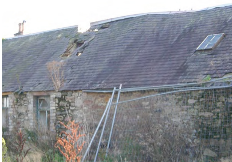
Plate 7: Building 2, north-west facing elevation
