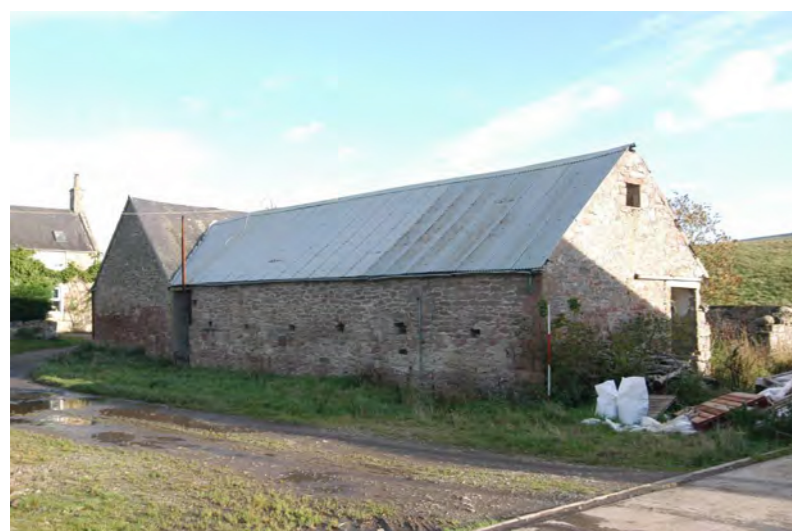
Plate 13: Building 3, Unit 3/1 byre north-west facing elevation
