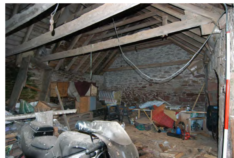
Plate 15: Building 3, Unit 3/2 interior detail
