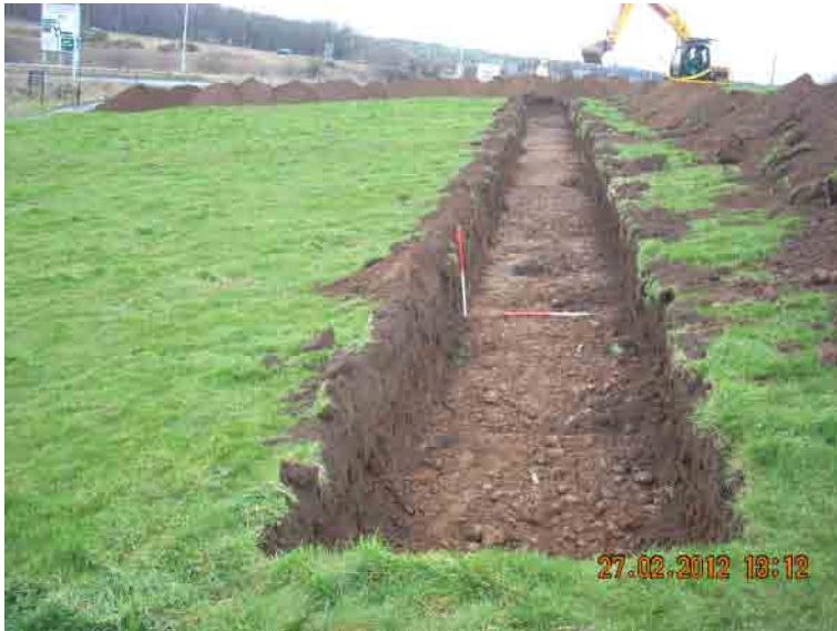
Fig. 2 General view of Trench 1
