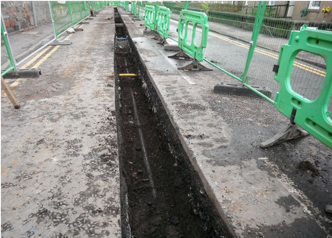
Fig. 3 - Cast Iron water pipe left in situ
