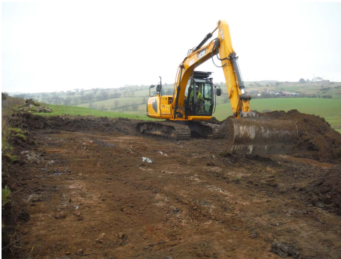
Fig. 4 - Photo of the area around the turbine base being stripped, from the SW
