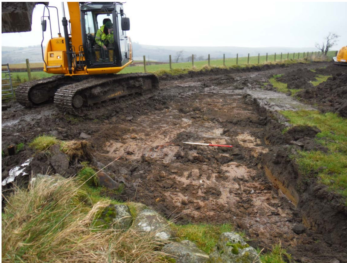
Fig. 5 - Photo of stripping the turning circle and revealing field drain 006/007, from the S
