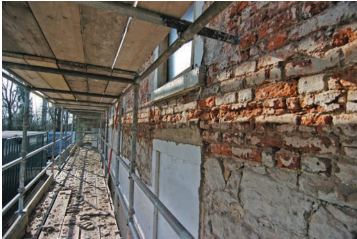
Fig. 37 - Exterior south-facing elevation, brickwork of the heightened East Wing
