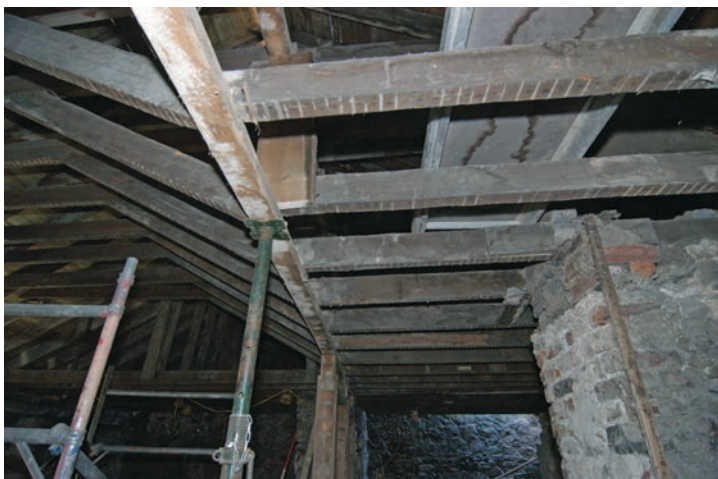
Fig. 31 - Unit 22 Supported A-frame trusses on former partition wall plate
