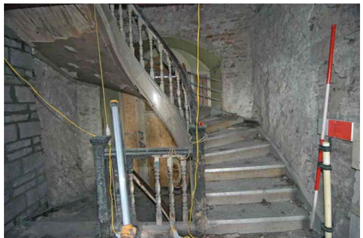
Fig. 26 - Unit 16, first floor stairs landing, main staircase detail
