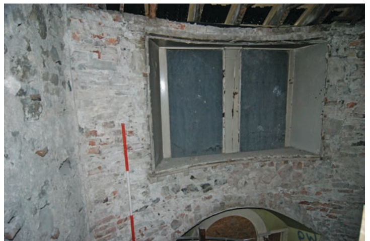
Fig. 32 - Unit 23, curving inserted stairs window and wall fabric detail
