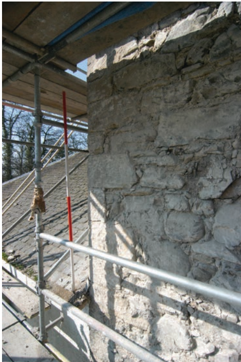
Fig. 35 - Exterior south elevation, quoins on the main block wall above the West Wing
