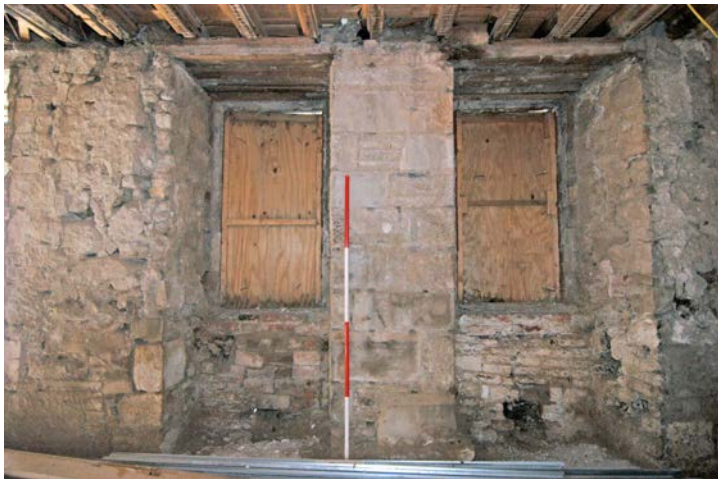
Fig. 12 - Unit 2, internal south wall (north-facing) splayed window detail
