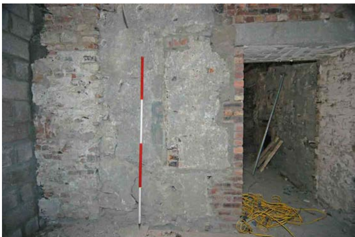
Fig. 25 - Unit 15, north-facing elevation, blocked chamfer-moulded window
