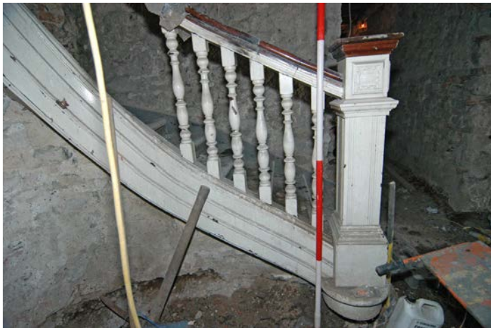
Fig. 18 - Unit 2 main staircase balustrade and handrail
