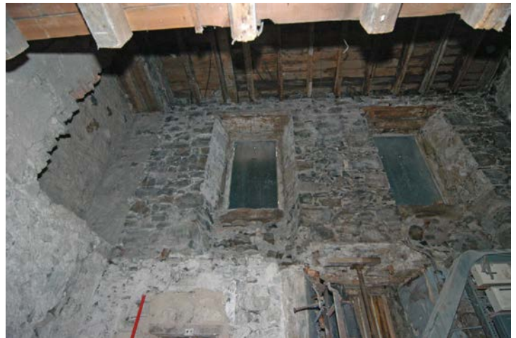
Fig. 19 - Unit 9 first floor level with first floor removed
