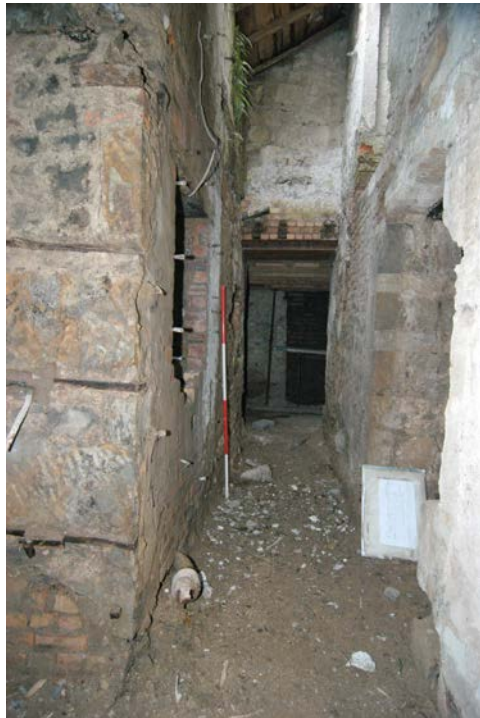
Fig. 16 - Unit 6 general view facing east after removal of partition walls
