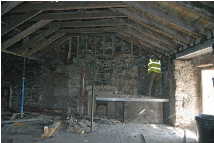
Fig. 29 - Unit 21, chimneybreast and roof trusses at the east end (west-facing elevation)
