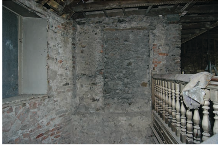
Fig. 34 - Unit 23 Blocked window (Fig 27) fabric detail and balustrade
