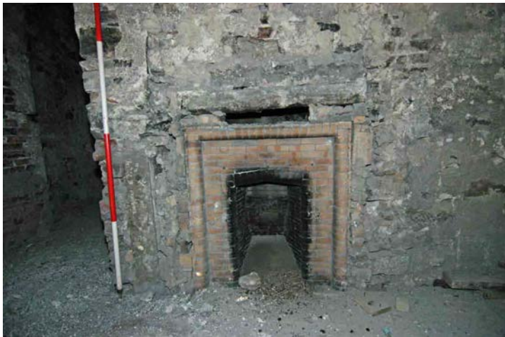
Fig. 23 - Unit 13, fireplace at the west end (east-facing elevation)
