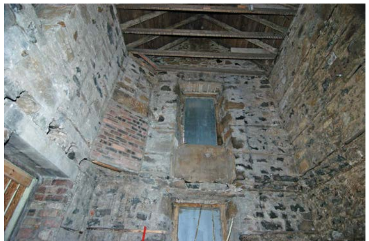
Fig. 15 - Unit 5 internal north-wall (south-facing) at first floor level fabric detail
