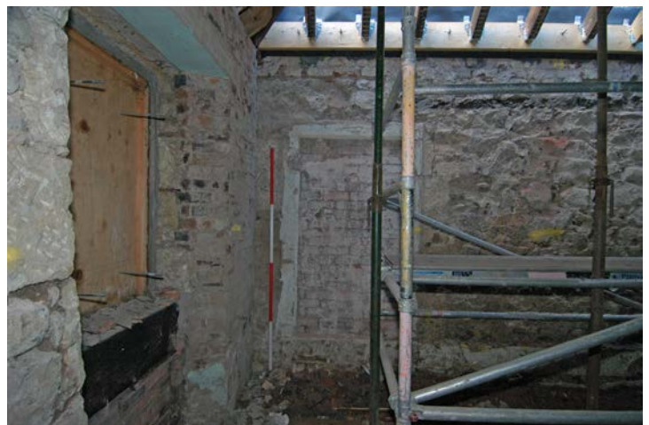
Fig. 20 - Unit 11, East Wing Blocked doorway with raised margins at ground floor
