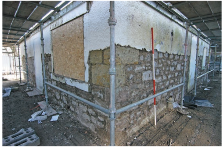
Fig. 38 - Exterior East Wing quoin detail following partial removal of the harling
