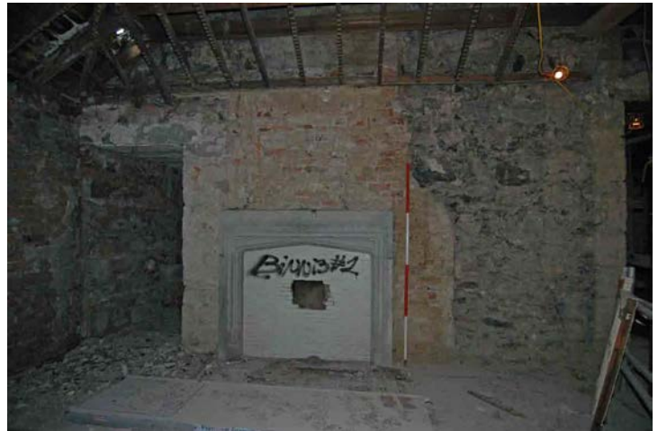
Fig. 22 - Unit 12, bedroom fireplace on the west wall, east-facing elevation
