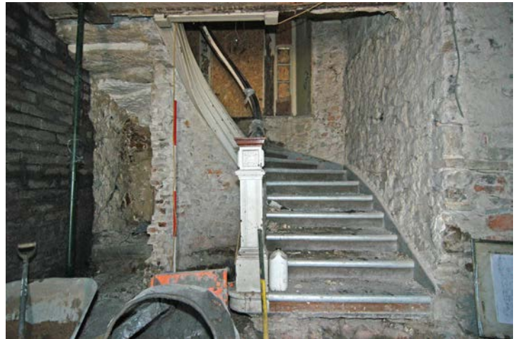
Fig. 17 - Unit 2 main staircase newel post and treads
