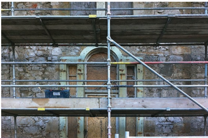
Fig. 39 - Exterior north-facing elevation showing quoins on either side of the Palladian window insert
