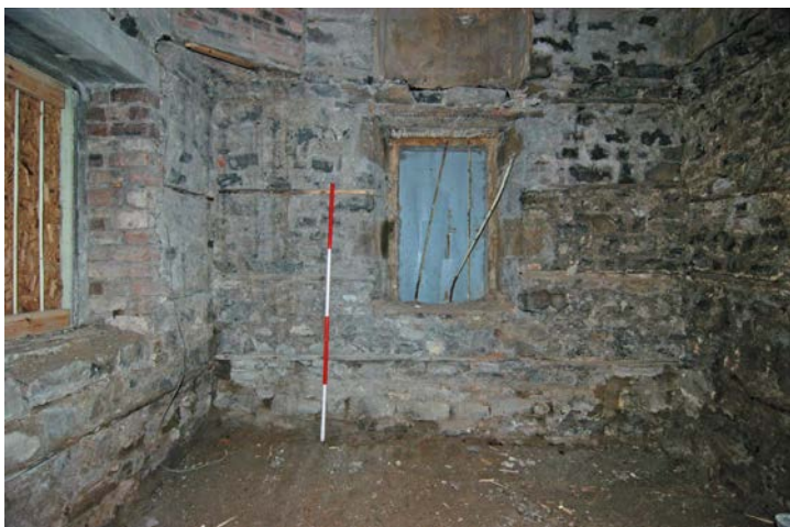
Fig. 14 - Unit 5 internal north wall (south-facing) fenestration and fabric detail
