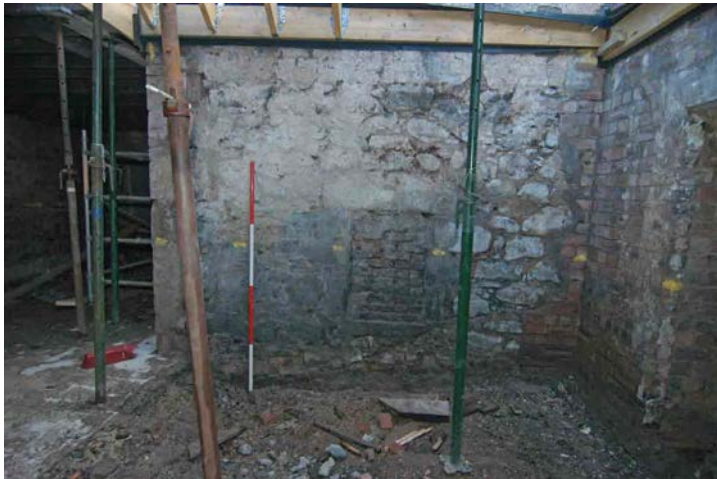
Fig. 21 - Unit 11, East Wing, blocked window with chamfer moulded surrounds
