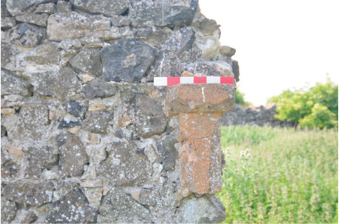
Fig. 5g - Detail of surviving pilaster on EFE south range
