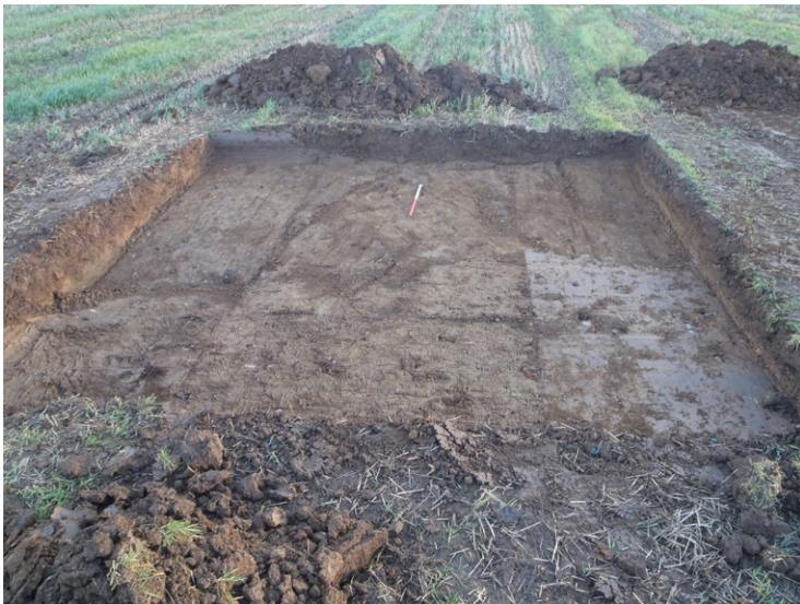
Fig. 4: Turbine 1 - Base Excavation
