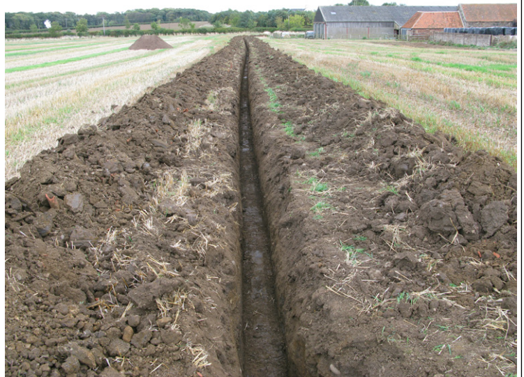
Fig. 3: Cable trench running SW to NE
