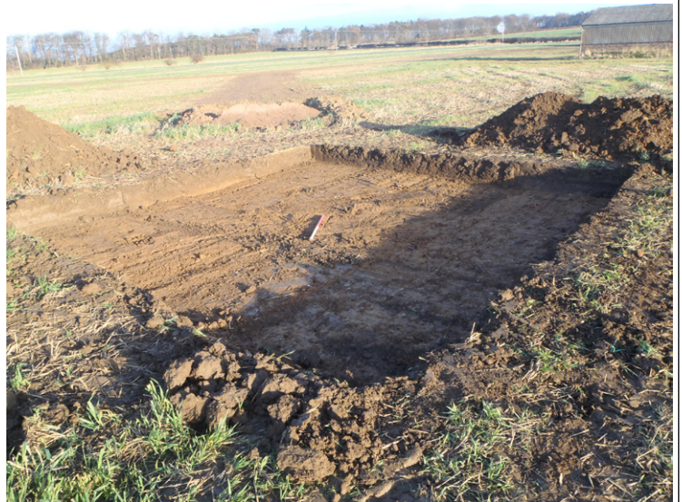
Fig. 5: Turbine 2 - Base Excavation
