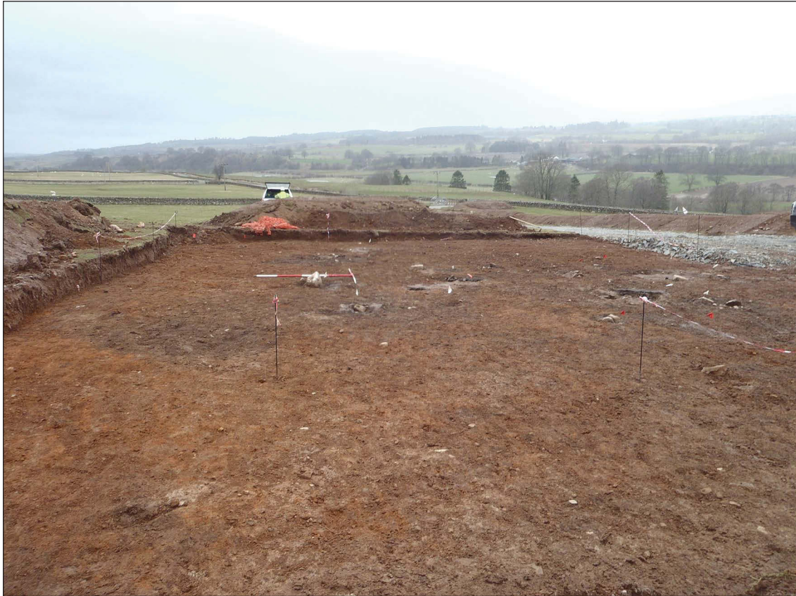
Fig. 8 – General view of excavation area at ZV230B
