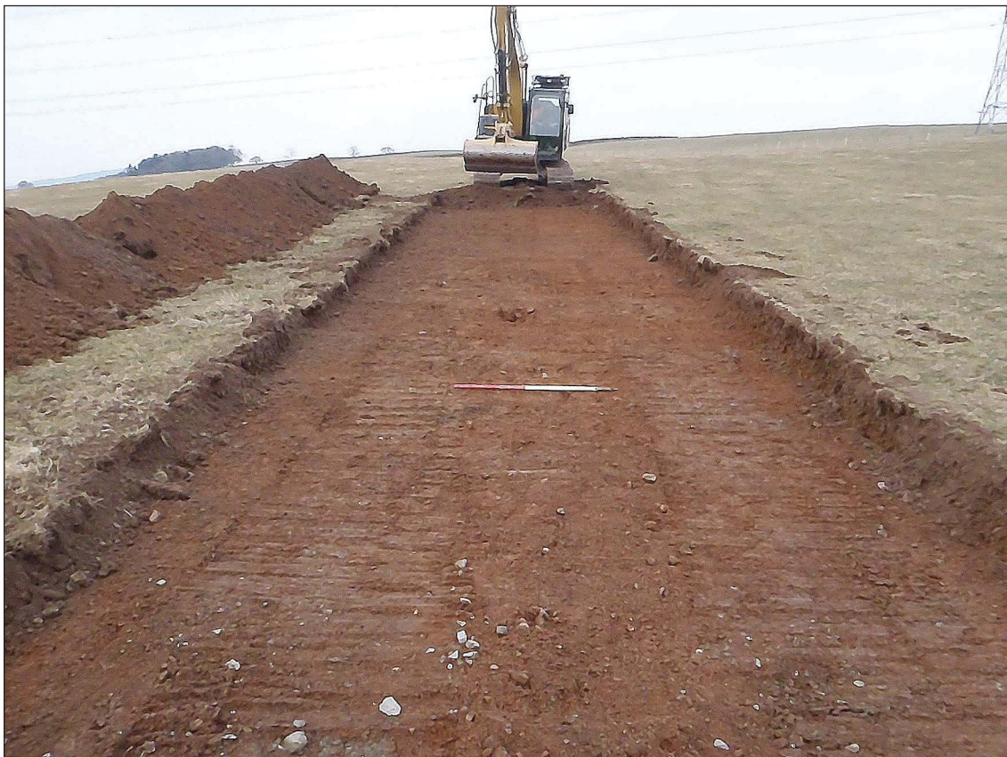
Fig. 7 – Access track to ZV230B
