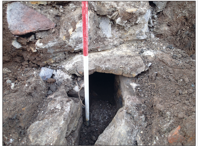
Fig. 3 - Box drain 004 in Tr 18
