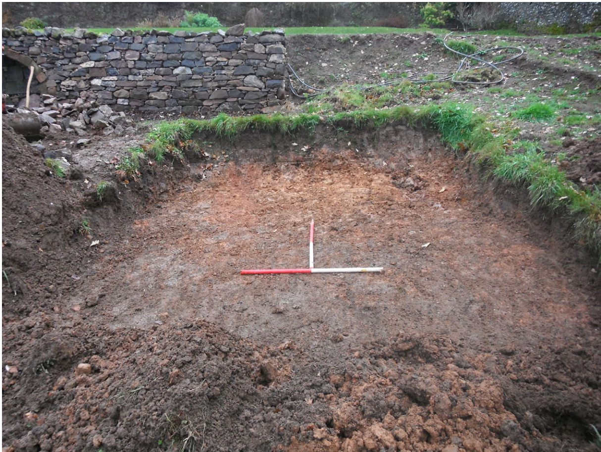
Fig. 2 - Development area from SW following soil stripping
