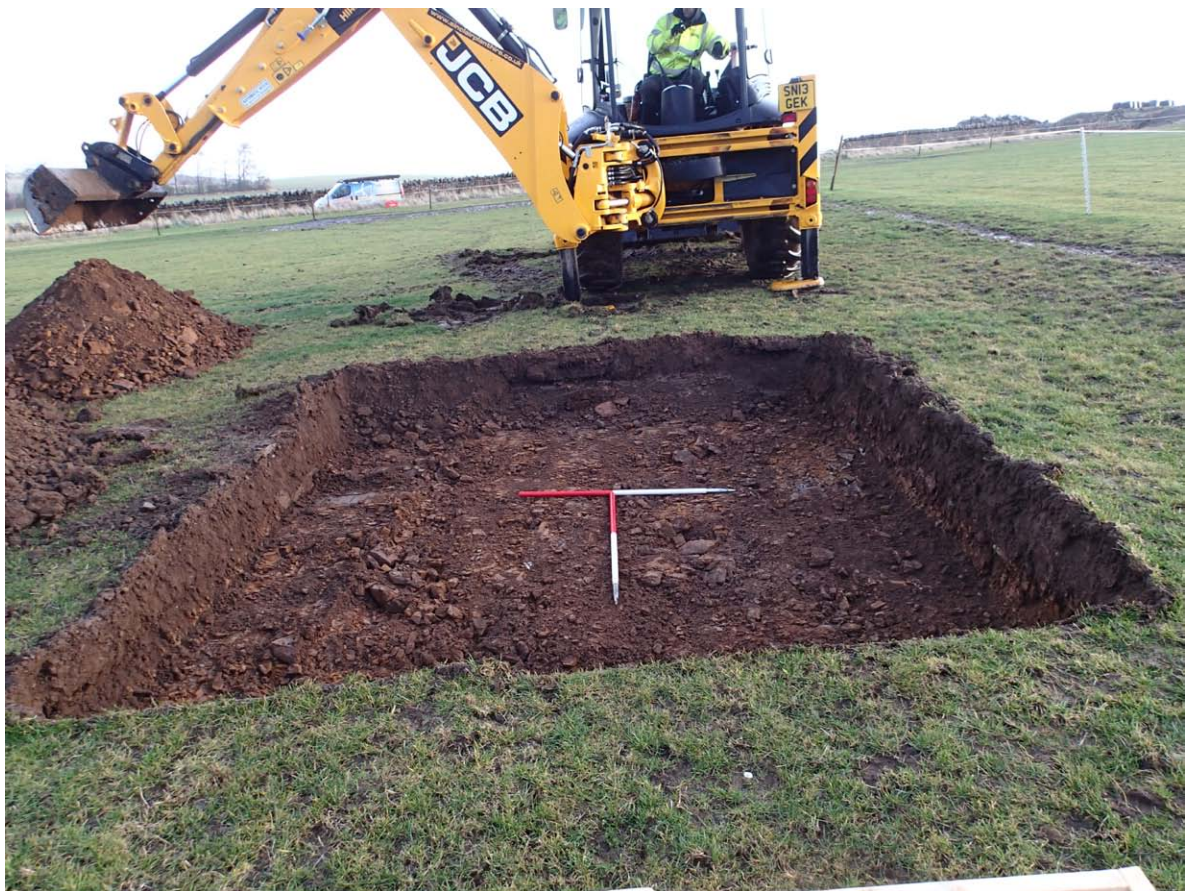
Fig. 3 - Turbine base excavated to natural subsoil
