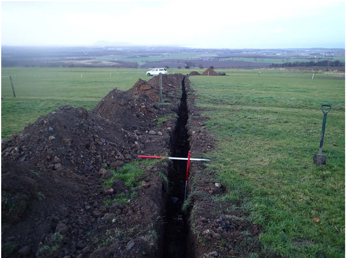
Fig. 5 - Line of cable trench looking NW
