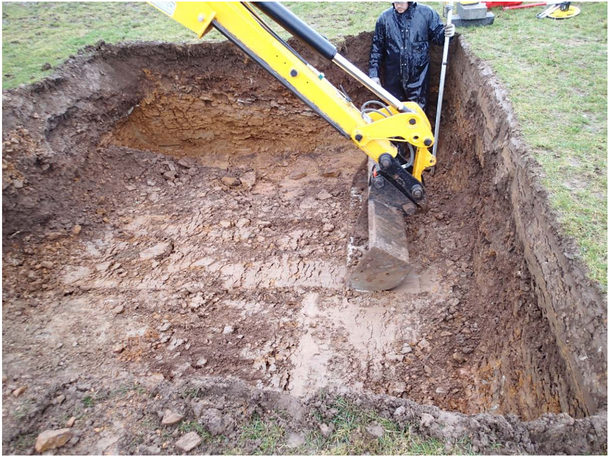
Fig. 4 - Turbine base excavated to full depth
