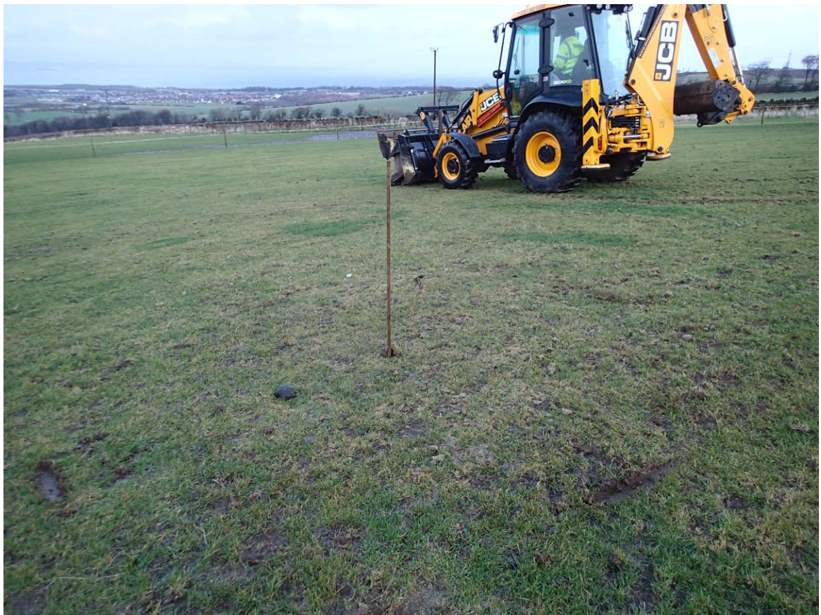
Fig. 2 - Turbine location pre-excavation
