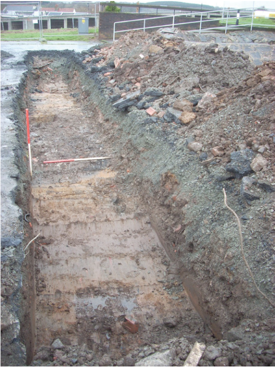
Fig. 7 - Trench 10, ditch (050) in the foreground with large circular feature (048) beyond from the south
