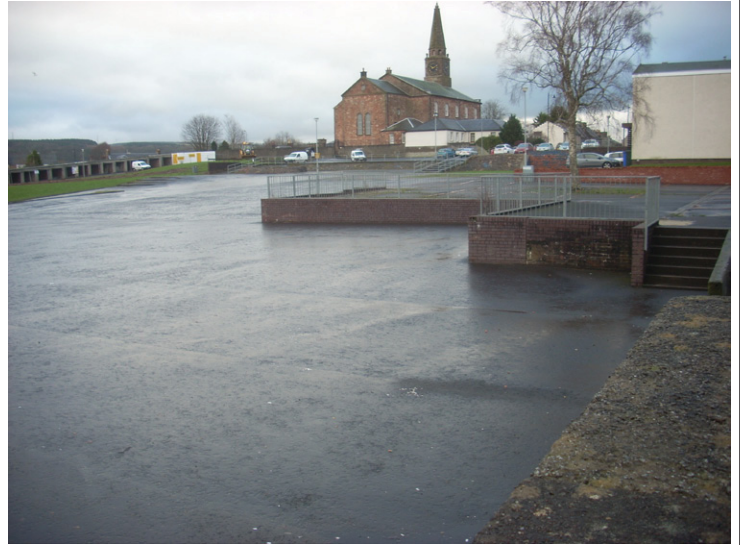
Fig. 4 - General view of the site from the south-west
