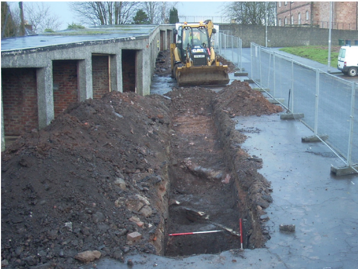
Fig. 5 - Trench 6, boundary walls 028, 029 and 030 from the west
