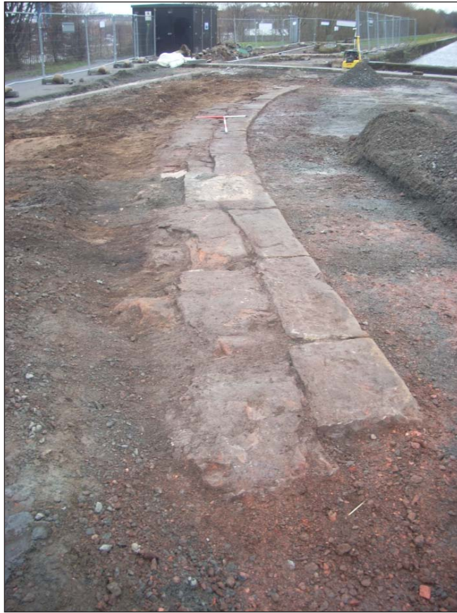
Fig. 4 - The original canal wall from the south
