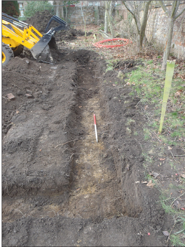
Fig. 4 - Northernmost foundation from the east
