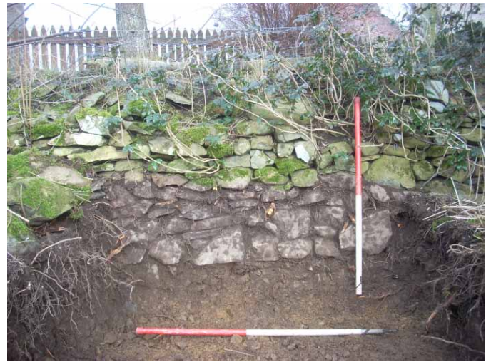
Fig. 3 - Trench 1, view of wall 001 constructed on natural subsoil
