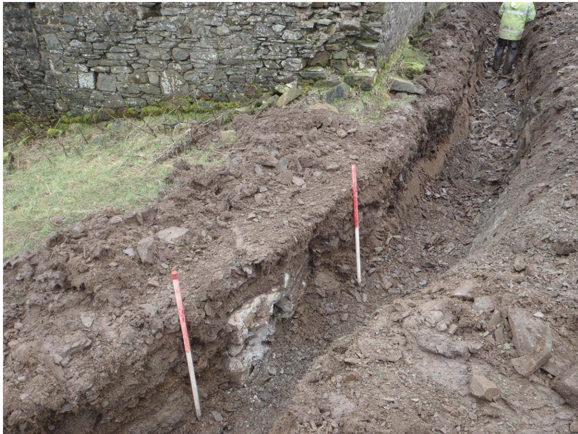
Fig. 4 - Foundations for the extension to Crawthat Cottage 008 revealed in trench
