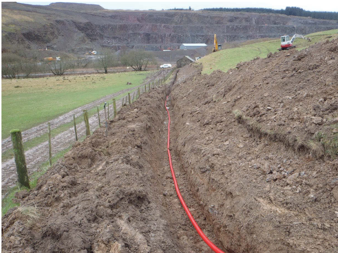
Fig. 5 - General shot of excavated cable trench to the SE of MDG7556
