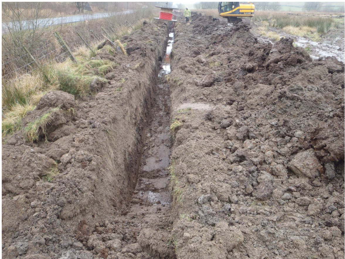
Fig. 2 - General shot of excavated cable trench next to the B7068
