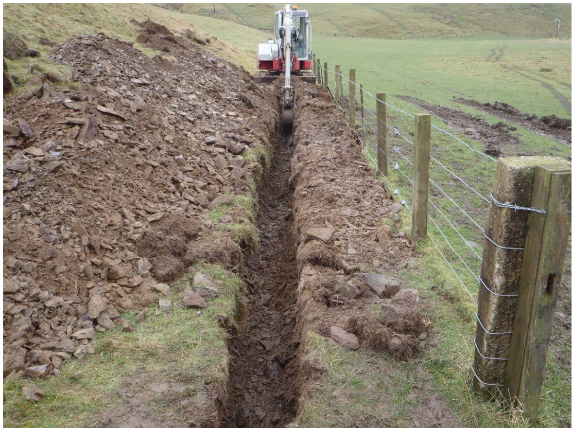
Fig. 3 - General shot of excavated cable trench SE of knoll
